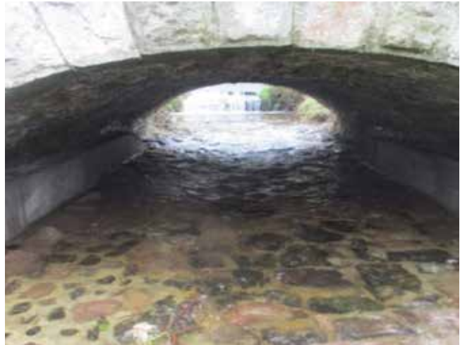
Pict 2.8 New bed and scour skirts installed
