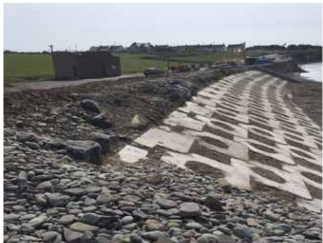
Pict.2.10 ECAB revetment in place at Garretstown beach
