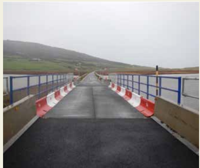
Pict 2.4 Road after temporary bridge installation
