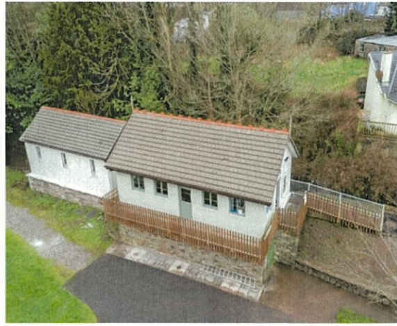
Figure 4-Refurbishment of Pitch & Putt Club, Town Park, Macroom
