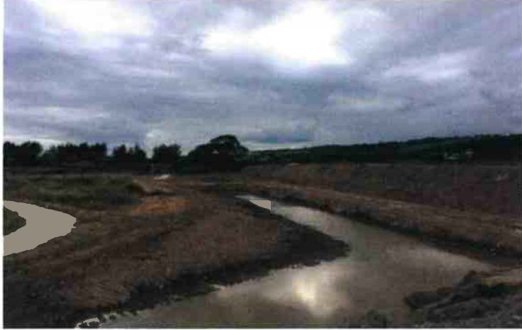
Installation of Nature Trail and Reed Bed at Harpers Island
