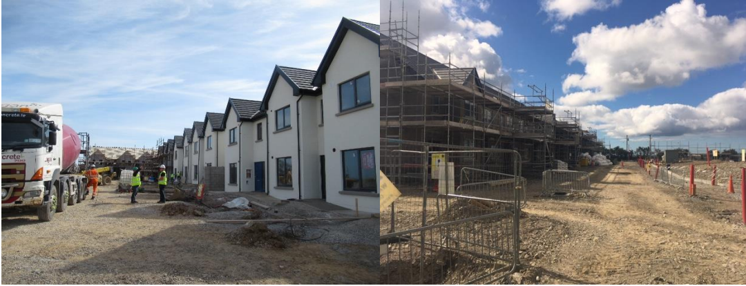
Units under construction in Youghal & Kinsale.
