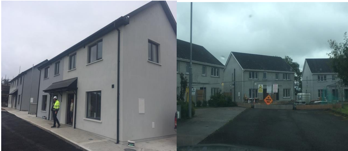
Completed houses in Doneraile and units under construction in Ballyhooley.
