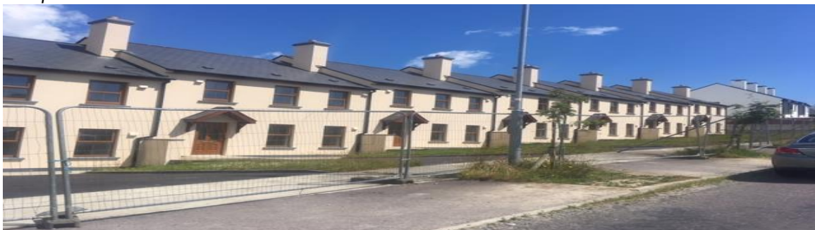
Completed units in Rosscarbery.
