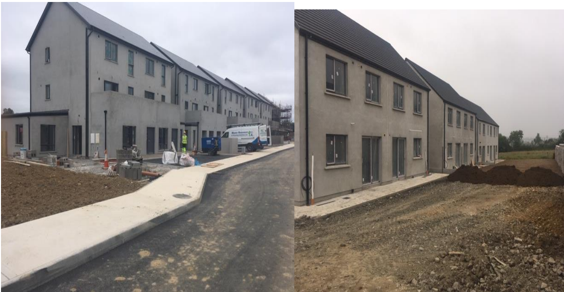
Houses under construction in Mallow & Kanturk.
