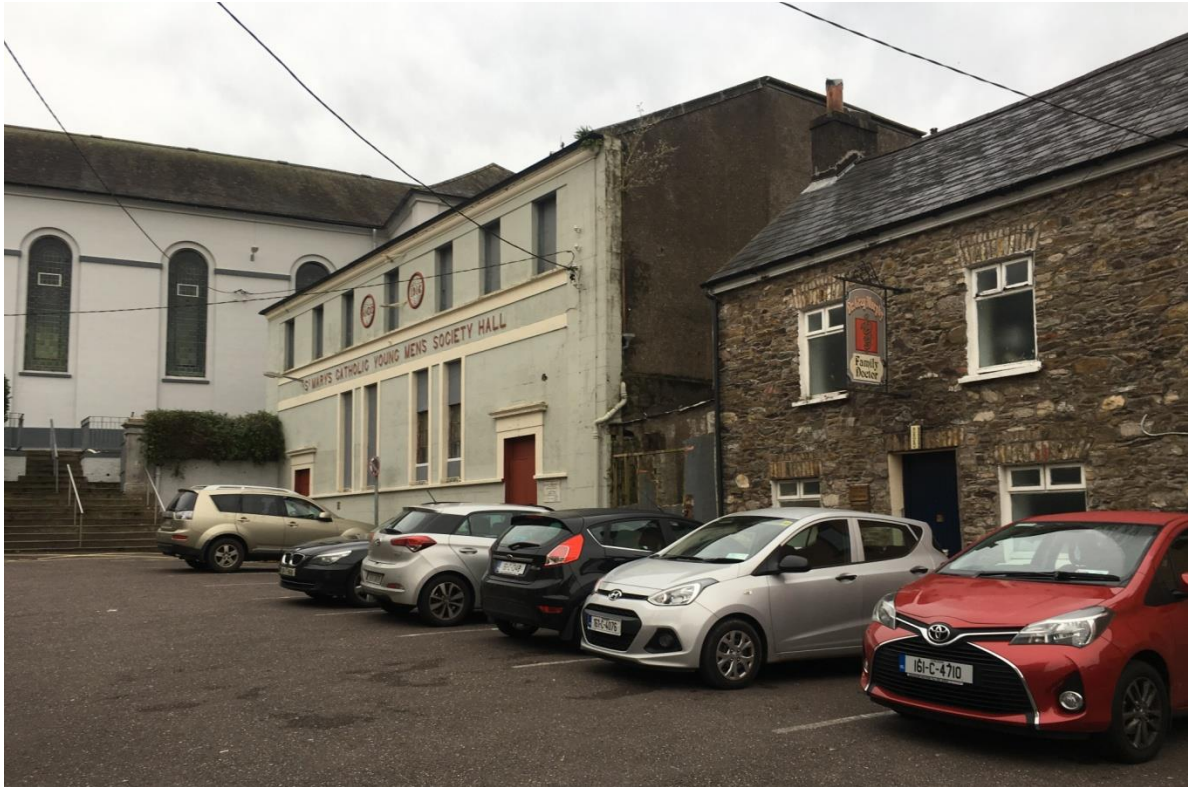
Fig.3.8 Streetscape of Passage West – Chapel Square
