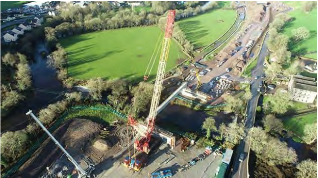
Figure 4.4.3: Contractors working on the N22 Baile Bhuirne Macroom by-pass
