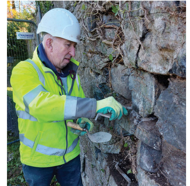
Repointing with lime mortar
