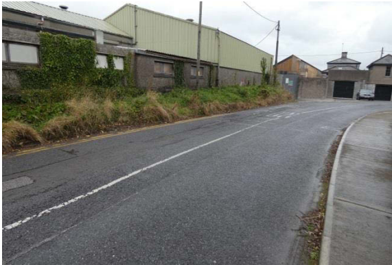
7(a,b) St Bernard's Place Embankment
