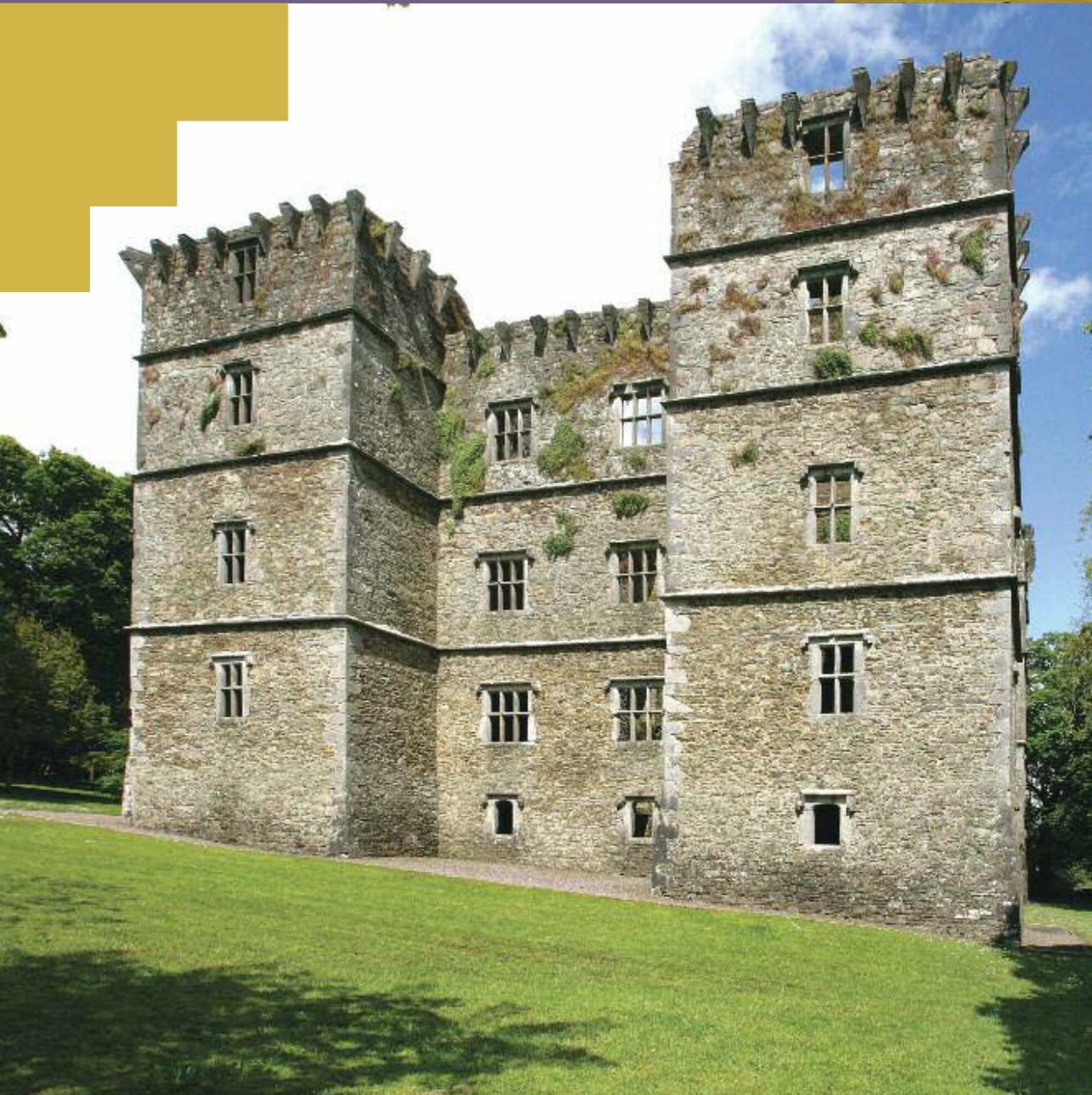
Kanturk Castle. Image courtesy of Tony Roche, National Monuments Service, Photographic Unit.
