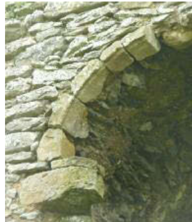
The surviving section of the half-round window at Ballyderown Castle.
