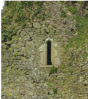
A typical simple ogee-head window.
