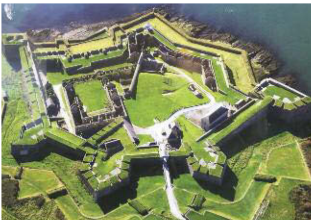
The 'star-shaped fort' at Charles Fort, near Kinsale. The projecting bastions are typical of seventeenth-century military fortifications.
