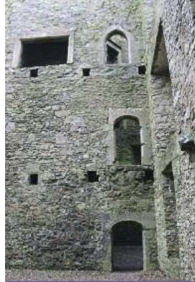
Internal doors at Kanturk Castle. Note the pointed arch on the upper door and the flatter Tudor arch on the two below.
