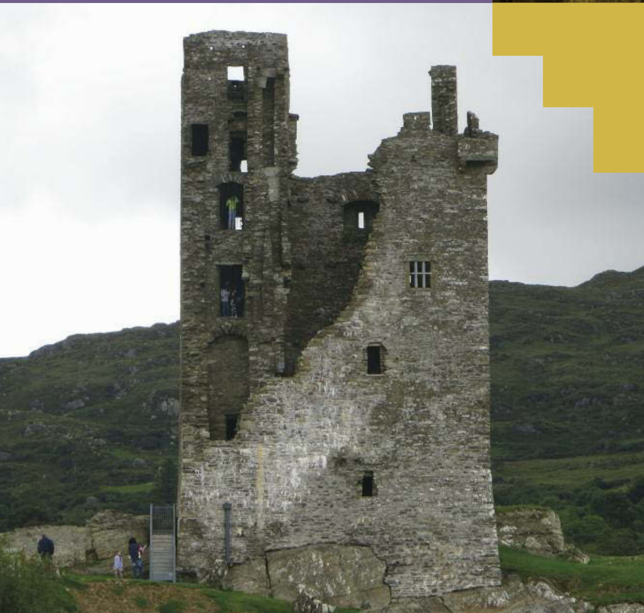
Castle Donovan from the south. The vertical series of small rooms and passages stacked directly above the entrance area is found in most Cork tower houses. To the right note the large lintelled window divided by vertical stone mullions and a horizontal stone tramson with projecting hood-moulding, typical of the late 16th and early 17th centuries.
