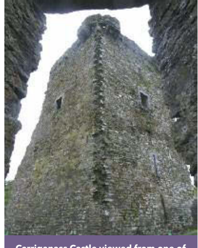
Carriganass Castle viewed from one of the bastions at the corner of the bawn wall. Note the extensive base battering.
