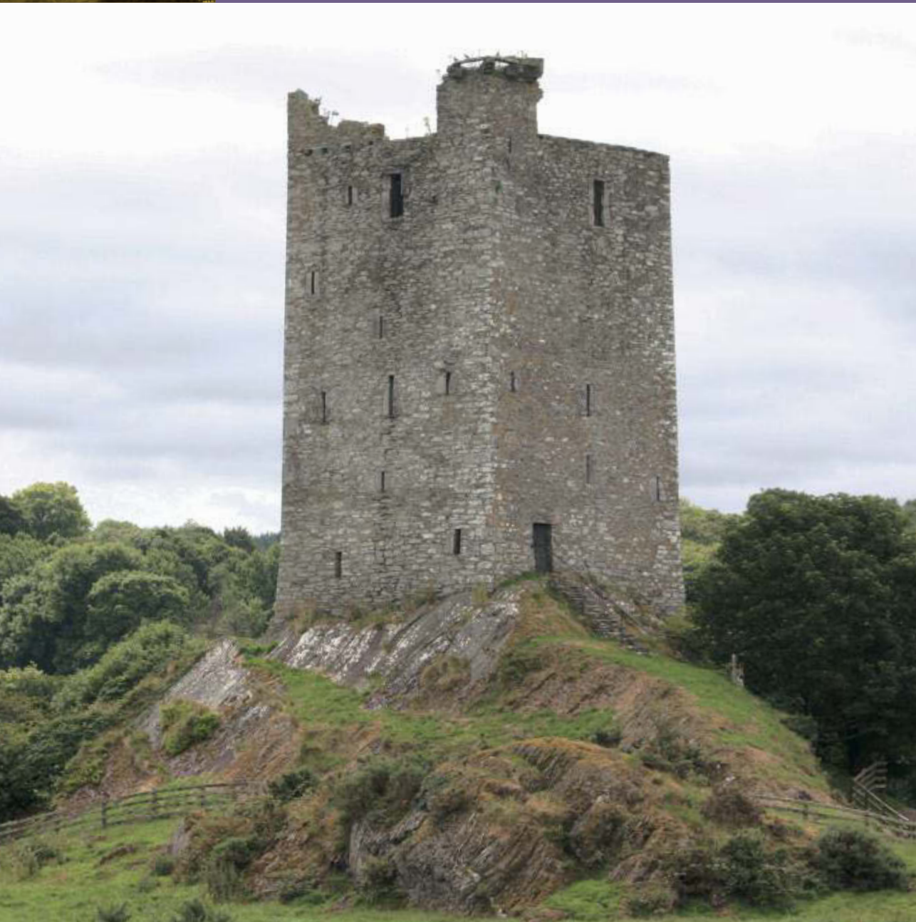
Carrigaphooca Castle from northeast showing steepness of approach to entrance doorway.
