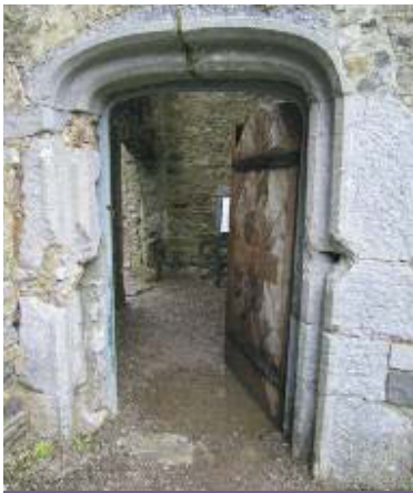
Mallow Castle entrance doorway, which has a flat arch (Tudor arch).
