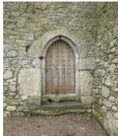
The pointed doorway to Barryscourt Castle. Note the roughly dressed limestone forming the doorway with 'yett-holes' at the apex of the arch and on the left-hand side.
