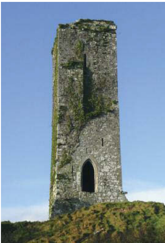
Ballincollig Castle watchtower with inserted 19th Century door with date plaque, 'W 1857'.
