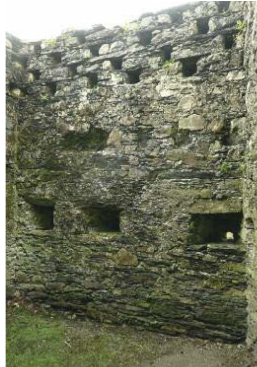
Interior view of flanking tower of seventeenth-century bawn at Carriganass Castle. Note gun loops at lower level and pigeon nesting boxes at upper level.
