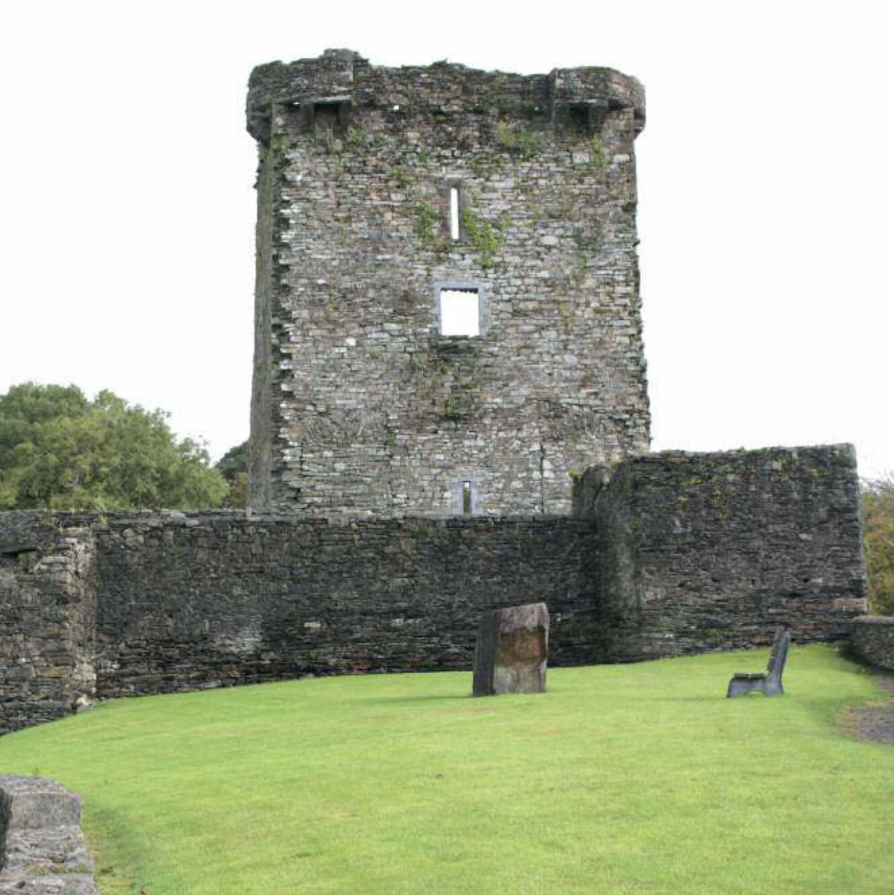
Carriganass Castle from the west. Note bartizans on wall tops. Also bawn wall in foreground.
