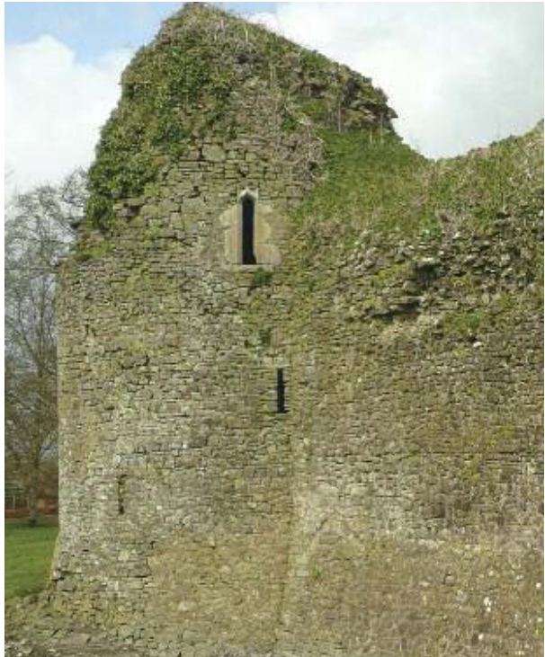
The west tower at Kilbolane. The ogee-head window near the top is part of a fifteenth-century rebuild.
