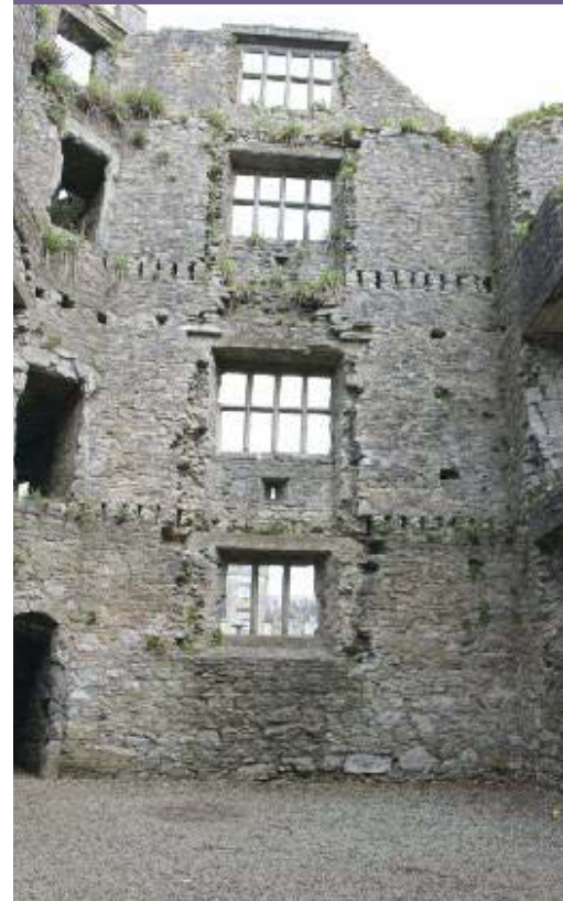
BELOW: Interior view of Mallow Castle. Timber floors throughout. Joist sockets are narrower and closed together than in earlier castles. Note gun loop between ground-floor and first-floor windows.
