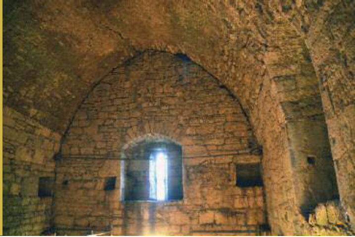
Belvelly Caslte - wicker centered vault on upper floor. Image courtesy of Dan Noonan.
