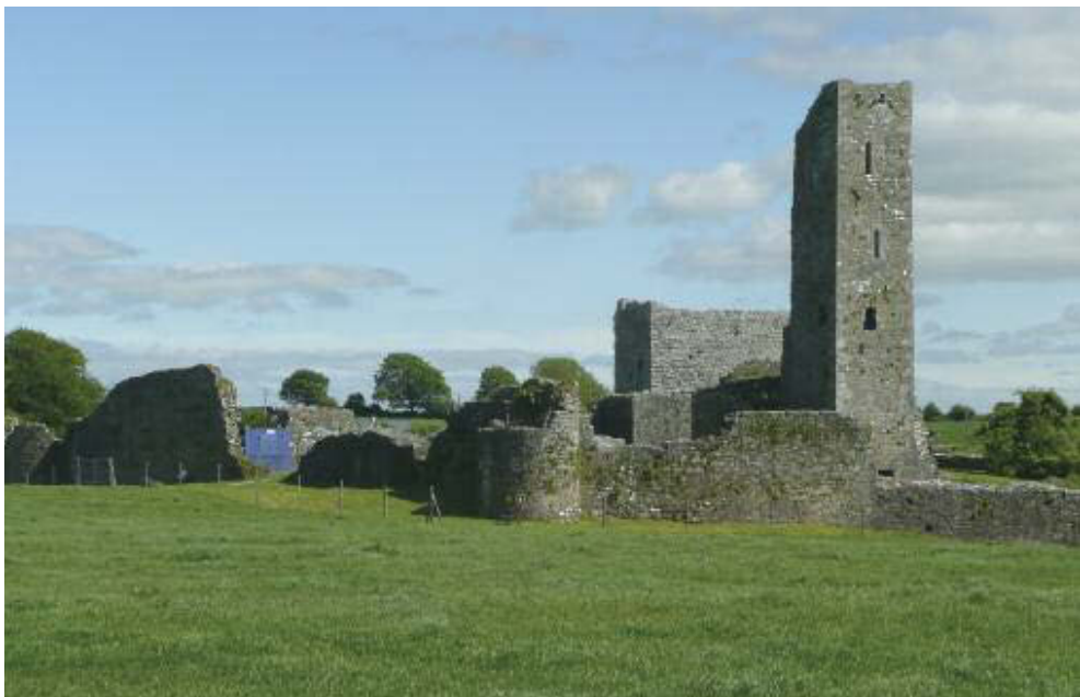
Glanworth Castle from the northwest. Curtain wall flanking tower in foreground. Gatehouse tower to right and chamber tower behind.
