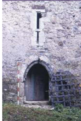
BELOW: The entrance door to Cregg castle. Note the iron 'yett' swinging open and the 'yett-hole' at the apex of the arch.
