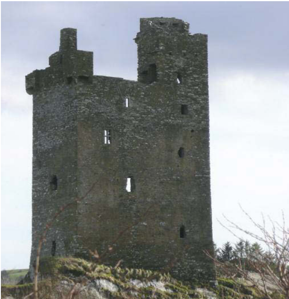
Castle Donovan from northeast. Note the large lintelled windows and bartizans on two corners.
