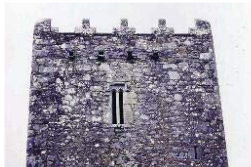
Drishane Castle with stepped battlements along parapet with projecting stone water spouts to drain water off wall-walk. A window with an elegant ogee head and hood moulding lights the Great Chamber within.
