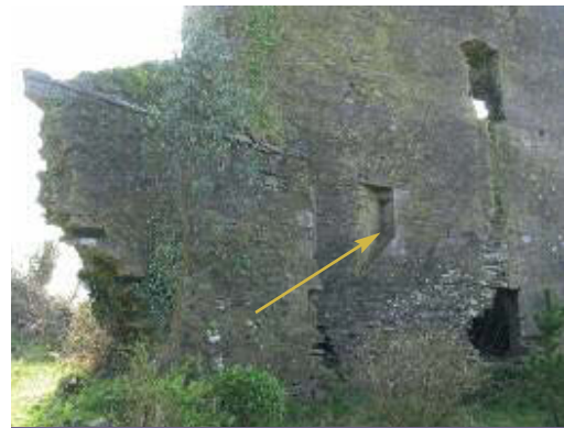
ABOVE: Angle bastion on corner of Mashanaglass castle. Note recessed gun-loop on castle wall.
