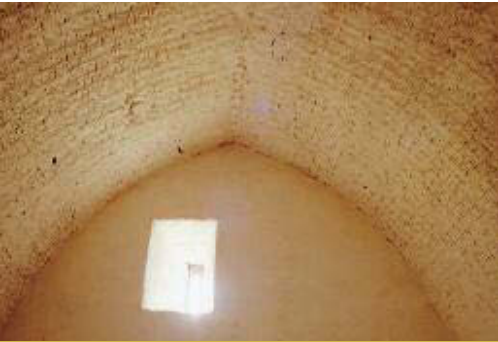
ABOVE: Wicker centred vault in Drishane Castle with imprint of wicker clearly visible in the plasterwork.
