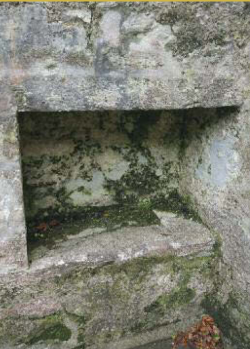
BELOW: A good example of a wall press, located on internal walls of a tower house for storage.
