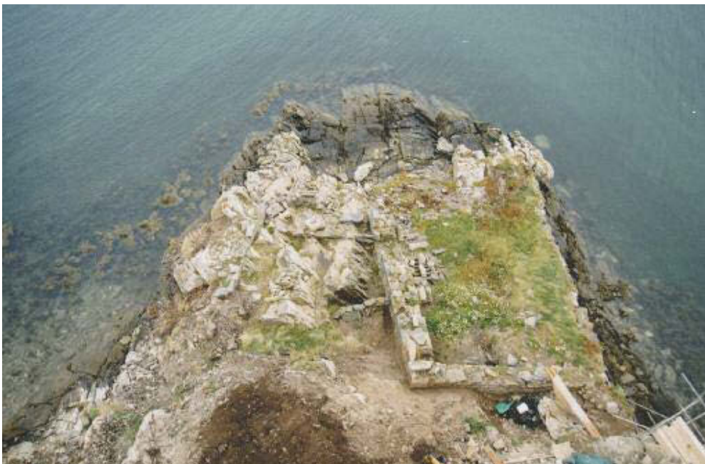
Kilcoe - aerial view of the building and slipway at the tip of the island on which the castle is built.
