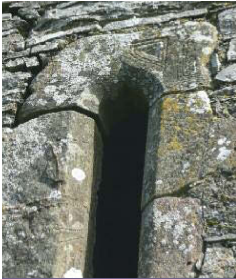
Ogee headed window at Ballinacarriga Castle with chamfered edges and decorative spandrels.
