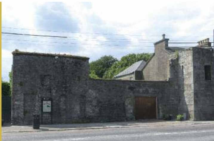
Lombard's Castle, Buttevant - the c. 15th/16th century urban residence for the Lombard family - merchants who originated from Italy and who were involved in the wool trade.
