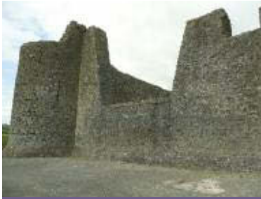
Flanking tower at Liscarroll Castle. Note the low base batter. The tall slit in the wall is a typical thirteenth-century arrow loop.
