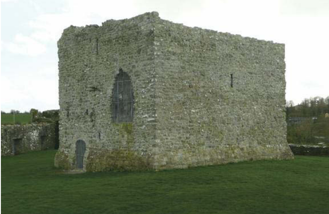
The 'chamber-tower' at Glanworth. The ground-floor door is not original. The larger opening on the first floor is the original entrance, which was reached by an external stairs. Note the base batter and the narrow window/arrow loops.
