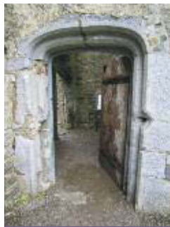
Mallow Castle entrance door, with flat 'Tudor' arch. Note yet-hole on right.
