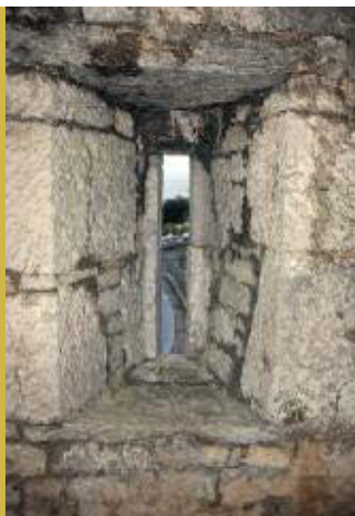
Belvelly Castle - Detail of window embrasure at Belvelly Castle with splayed ingoings. Image courtesy of Dan Noonan.
