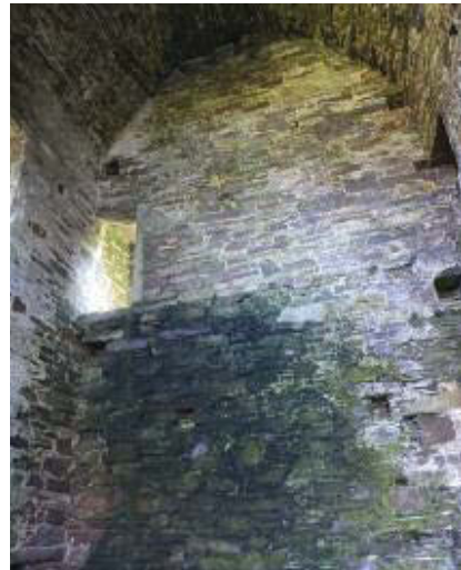
Vaulted ceiling of Dunmanus Castle. Access through door is from above.
