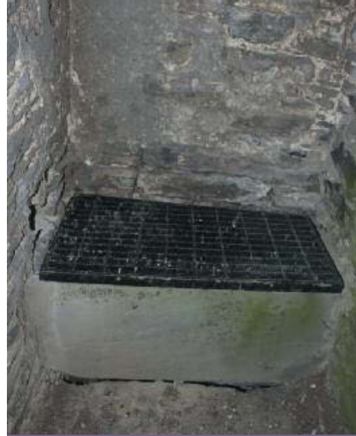
ABOVE: The garderobe at Carrigaphoooca castle. A wooden toilet seat would have been where the iron grille is now.
