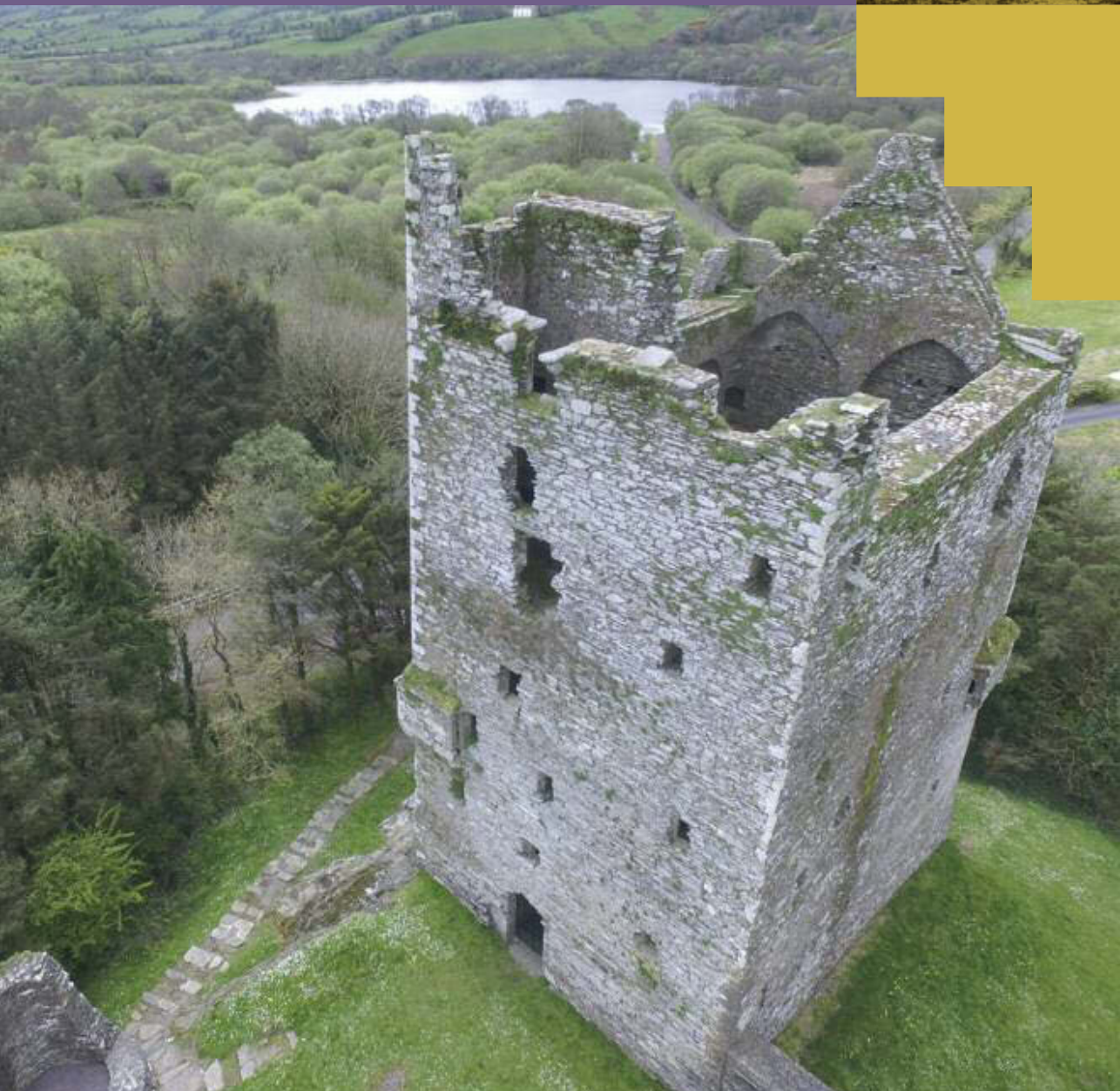
Ballinacarriga Castle from the air. Inside note decorative arcading in the Great Chamber on the top floor. Lower left of photo remains of circular corner tower on bawn wall. Also note bartizans on left and right corners of castle. Image courtesy of Margaret Hurley.
