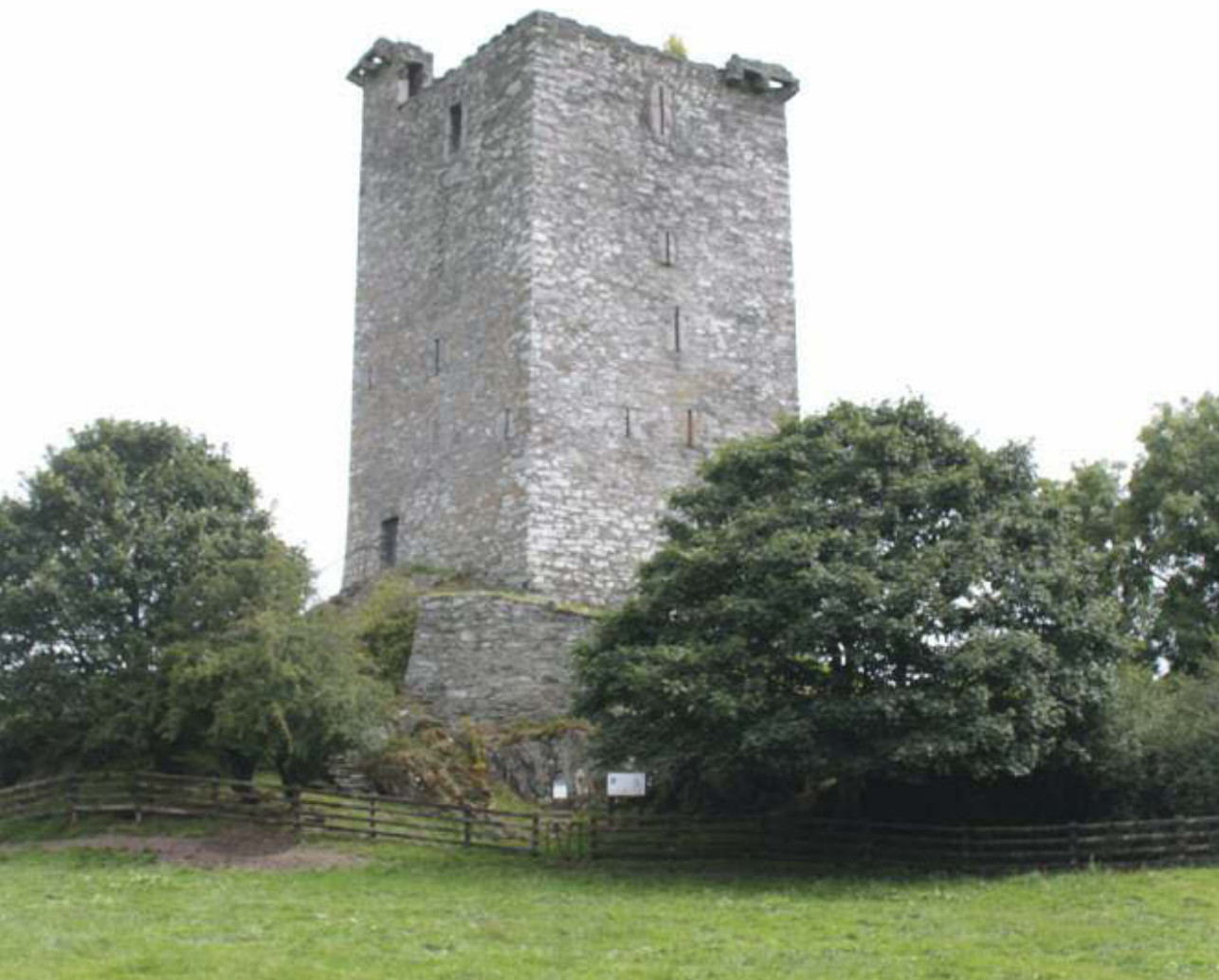
Carrigaphooca castle from the west showing remains of bartizans on two corners.
