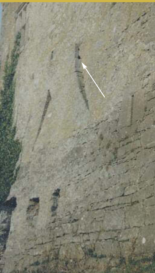
BELOW: Ballynamona castle, side view of one of the gun-loop recesses.
