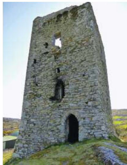
Dunmanus Castle - note the ground floor entrance and raised entry, first floor.
