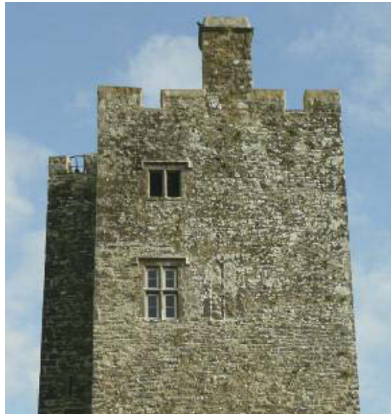
Seventeenth-century windows in Ballyhooly Castle. Note the transoms and mullions dividing the lower window. Also the projecting 'hood-moulding' over the windows. To the right of the lower window an earlier blocked-up double 'lancet' window can be seen.
