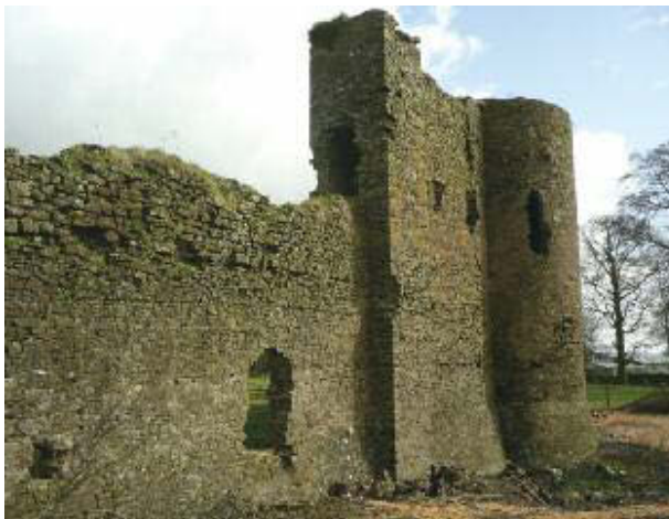
The south tower at Kilbolane. Note the door leading onto the wall top and the base batter near ground level.
