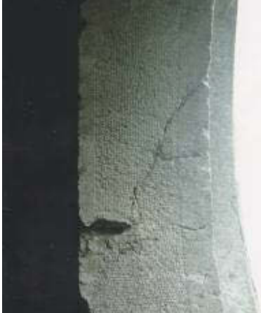
Punch dressing with drafted edging on the underside of the door arch at Ballynamona Castle.
