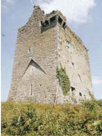
ABOVE: Ballynamona castle, with the gun loop recesses in the walls and bartizan overhead on the corner, clearly visible.
