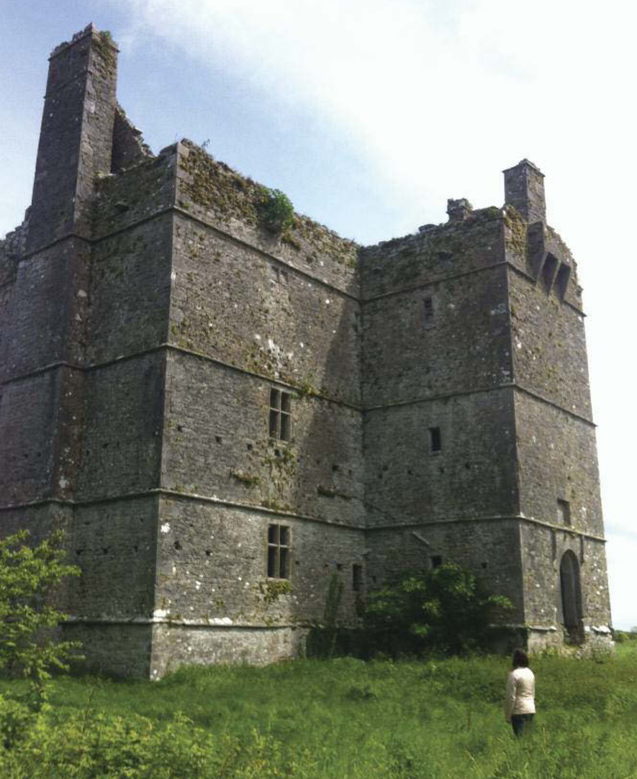
Ightermurragh fortified house. Note the machicolation above the door, which is more typical of a tower house than a fortified house.
