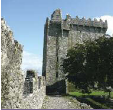
Blarney Castle stepped battlements and continuous machicolation (location of the famous Blarney Stone).
