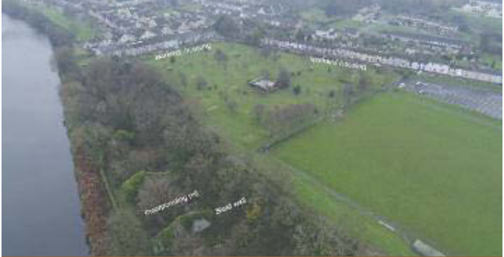
Aerial view of incorporating mills at Ballincollig Gunpowder Mills Complex, looking east.
