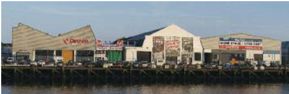
The location that the Ford Motor Works occupied on the Marina in Cork City.
