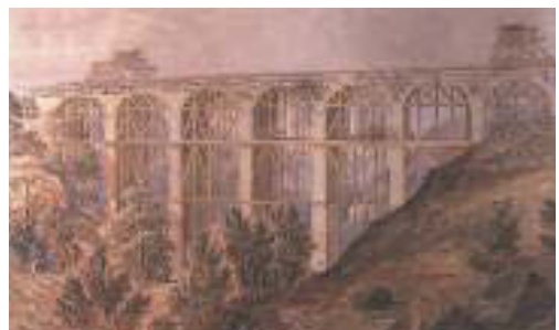
Great Southern & Western railway viaduct under construction over the Monard Glen, in 1846. Watercolour by R. L. Stopford, courtesy of the Crawford Art Gallery, Cork.
