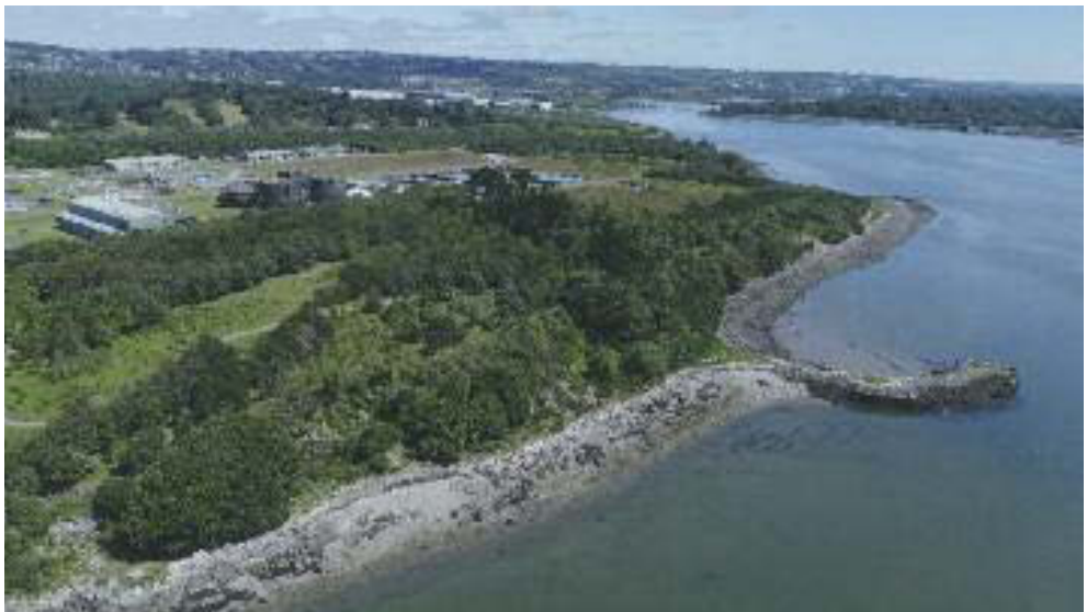
Carrigrenan quarry adjacent to the coast with jetty, the quarry mainly supplied ballast for ships.
