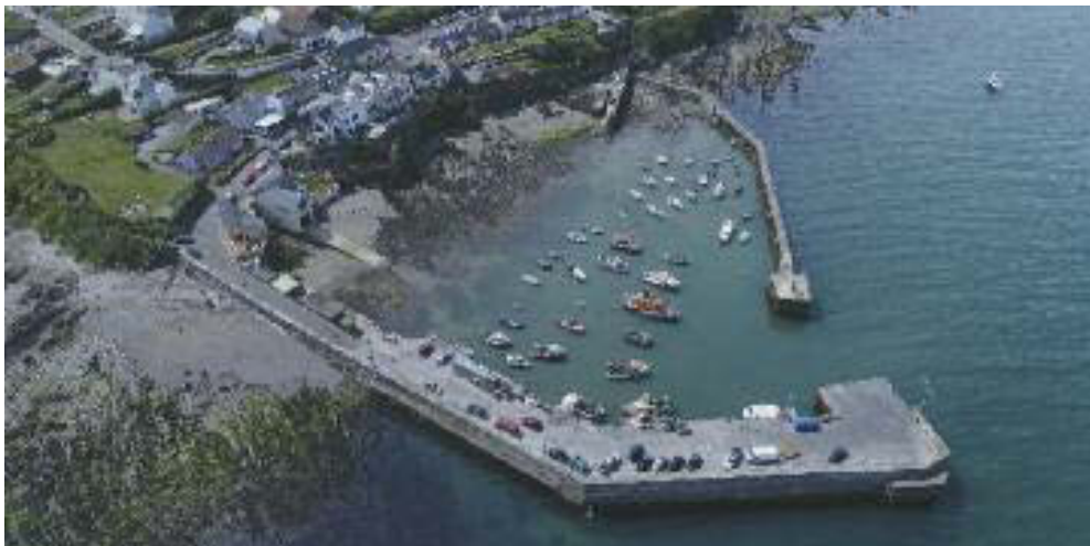
Aerial view of pier and breakwater at Ballycotton.
