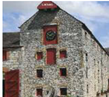
Sack hoist and lucamb, and loading doors for individual floors on grain store of c. 1825, at Midleton Distillery. Note the use of brick dressings (made with clamp-fired brick), and the painting of loading doors and window shutter with red lead paint.
