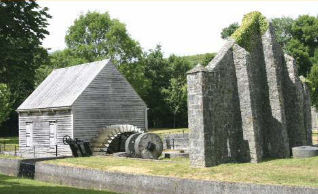
Restored incorporating mill (No. 1) c.1999 at Ballincollig Gunpowder mills with pair of edge runner stones adjacent to waterwheel and blast wall.
