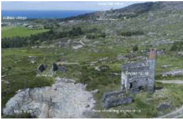
The engine house at the Coom mine, Allihies, c. 1871, powered the winding machine. Note the Mountain Mine in the background.
