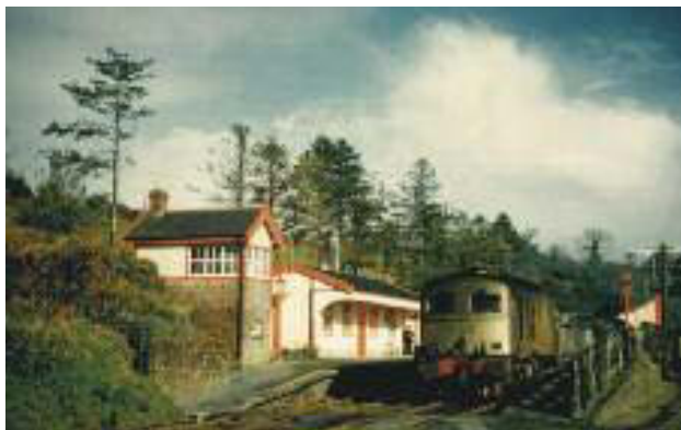
Ballinhassig Railway Station, closed 1961. (John L. O'Sullivan).
