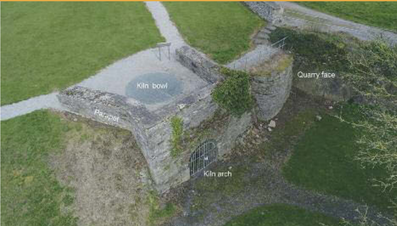
Castlelyons limekiln built into a slope to facilitate charging.
