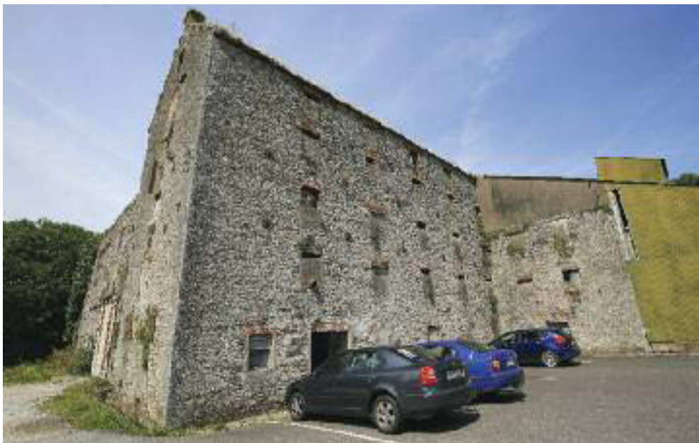
View of Killeagh Mills, from courtyard, showing current use as car park.
