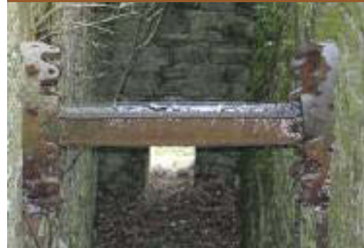
BELOW: Axle of the suspension waterwheel (c. 1802) at Overton Cotton Mills, near Bandon. It is the earliest known example of Suspension waterwheel in Ireland.
