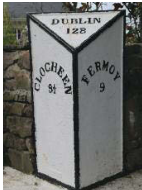
Cast iron turnpike milepost on the Cork-Dublin turnpike.
