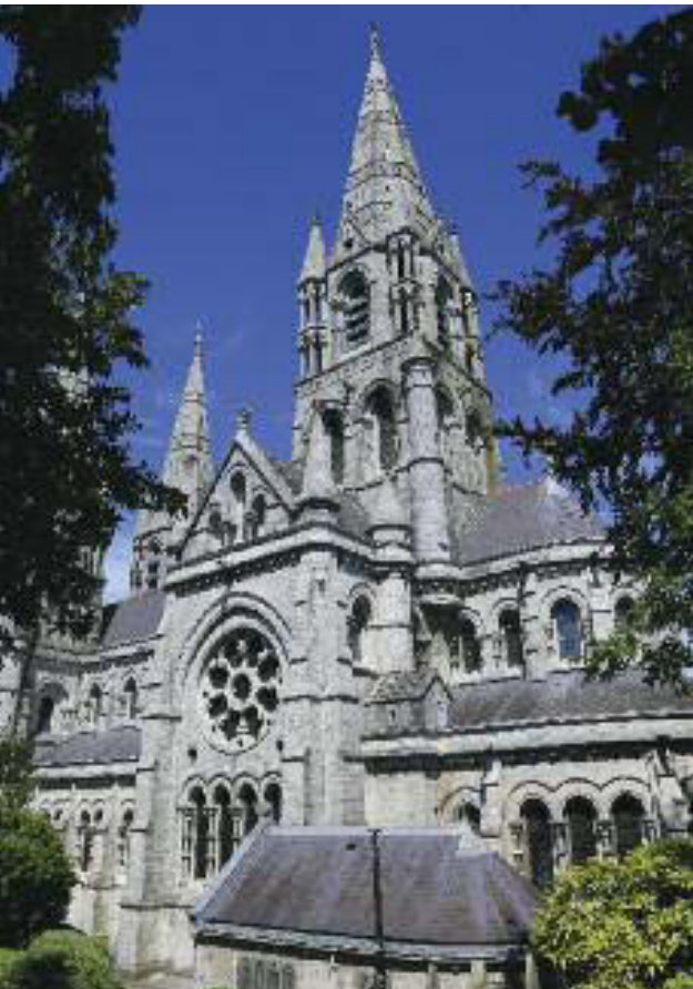
St Fin Barre's Cathedral, Cork, built between 1865-79 with stone from the Carrigmore quarries near Blackrock.
