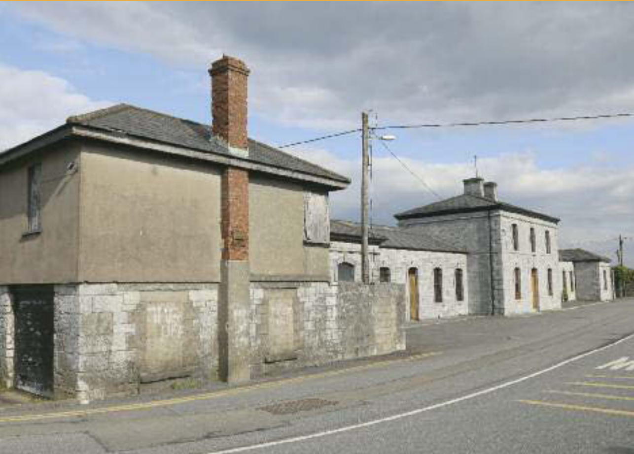
Fermoy railway station (1860), terminus of the Mallow-Fermoy railway.
