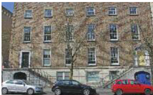
Buildings with imported Dutch brick façades on the South Mall, Cork City.
