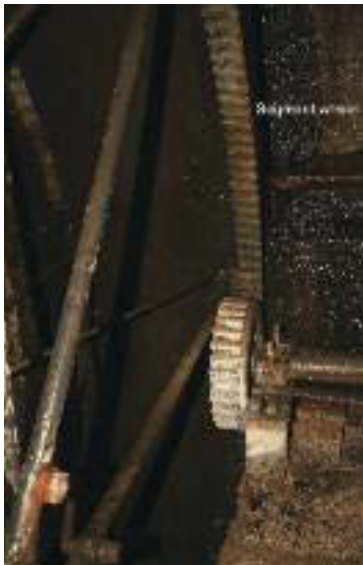
Suspension waterwheel with the segment wheel attached to the outer rim of waterwheel and smaller pinion wheel or bull nut transmitting power into the building, c. 1829, at Dyan Mills, county Tyrone.
