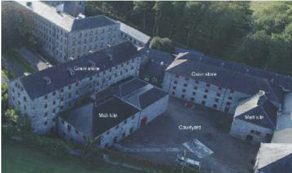
Midleton Distillery, showing grain stores and malt kilns arranged around a central courtyard, to facilitate vehicular access.
