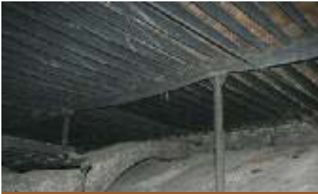
Interior of malt kiln at Midleton Distillery. The furnace was in the centre of the ground floor and the grain was laid on the brick tiled first floor. The weight of the grain and the tiled floor was substantial and needed the support of cast iron stanchions. The tiles had several perforations, allowing heat from the kiln to pass through and thus dry the grain.
