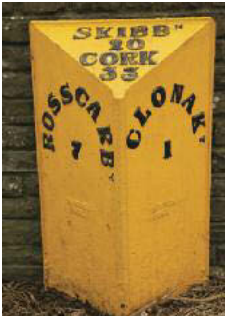
Cast iron milepost, made at the Barnes foundry on Hanover Street, Cork City (later the Hive Iron Foundry) in the 1820s, and erected by the Cork Grand Jury on the Cork-Skibbereen mail coach road outside Clonakilty.
