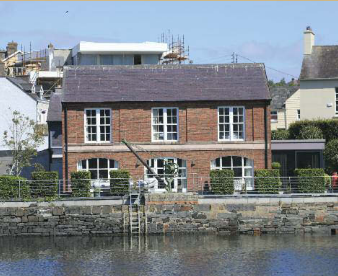
Fish store of c. 1860, at Scilly Point, Kinsale. Up to quite recently the windows on this building were louvred. A cast-iron crane, for unloading boats can be seen on the quayside.
