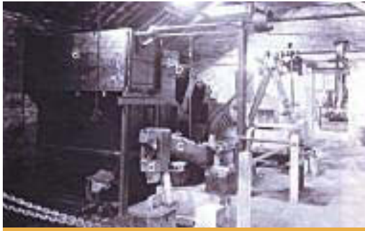
Interior of Logwood Mill at Monard in late 1940s: a. Feeder cistern with shuttle; b. High breastshot water with clasp arms, c. Trip hammer; d. Hammer head.
