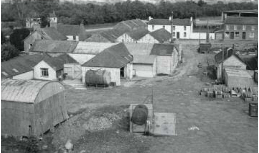
The presence of corrugated iron roofing can be seen on many of the buildings located within the Lombardstown Coop and Creamery, circa 1892. Image courtesy of Donie O'Sullivan.
