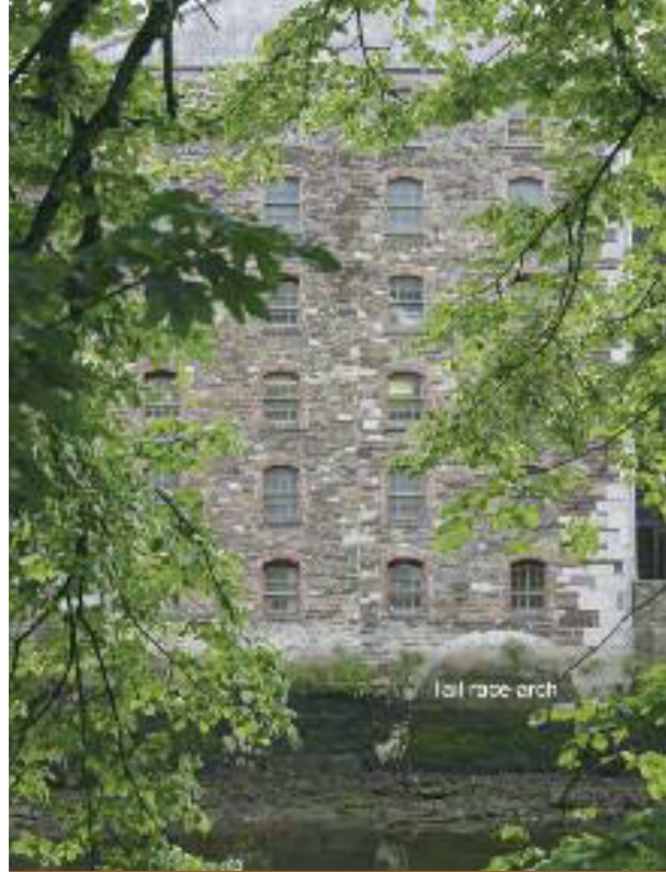
Brick dressed windows at Lee Mills, Cork City, completed between 1824 and 1832. Tail race arch and quoins of cut grey limestone in contrast with random rubble red sandstone walls.
