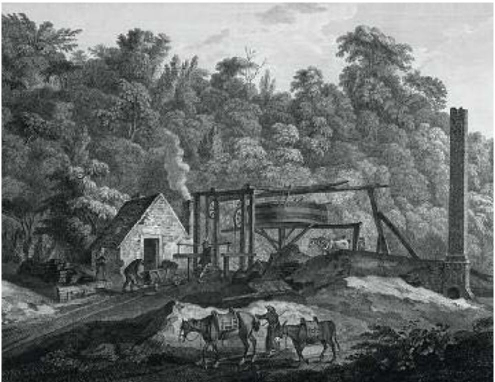
Horse whim in use at coal pit at Brosely, Shropshire, England in 1788.
