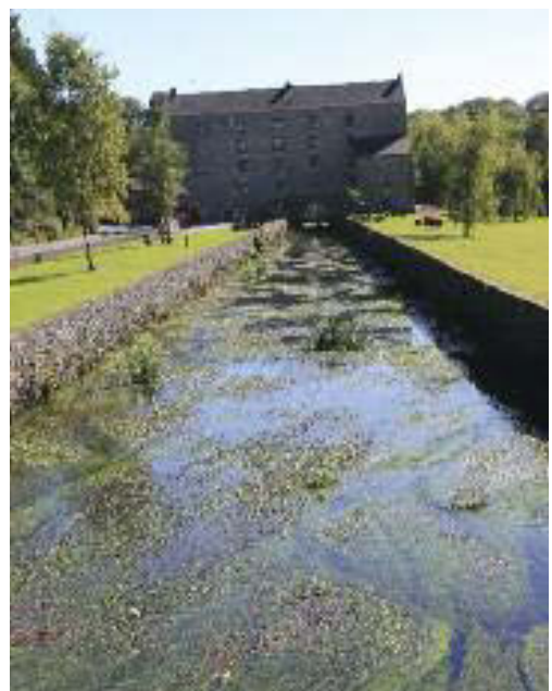
General view of 1820s millrace at the Bridge Mills Castletownroche, leading to arched waterwheel emplacement.
