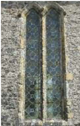
Yellow Dundry stone used in window dressings at St Colman's Cathedral, Cloyne.
