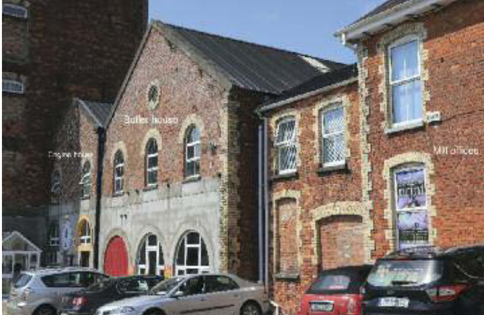
Engine house and boiler house at Donnybrook mill, Douglas. The three arches on the boiler house suggests that it originally housed three boilers.
