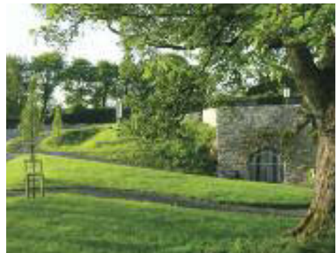
Limekiln as viewed from the south.
