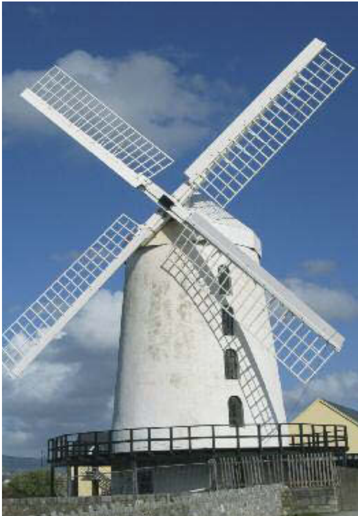
Reconstructed early nineteenth-century multi-storey tower mill at Blennerville, county Kerry.
