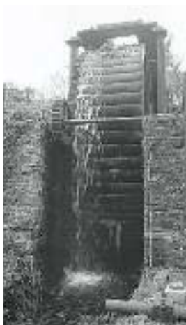
Overshot Suspension waterwheel at Dromore Mill near Dunmanway (Cork Archaeological Survey 1985).
