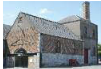
The building housing the 1826 pot still at Midleton Distillery.
