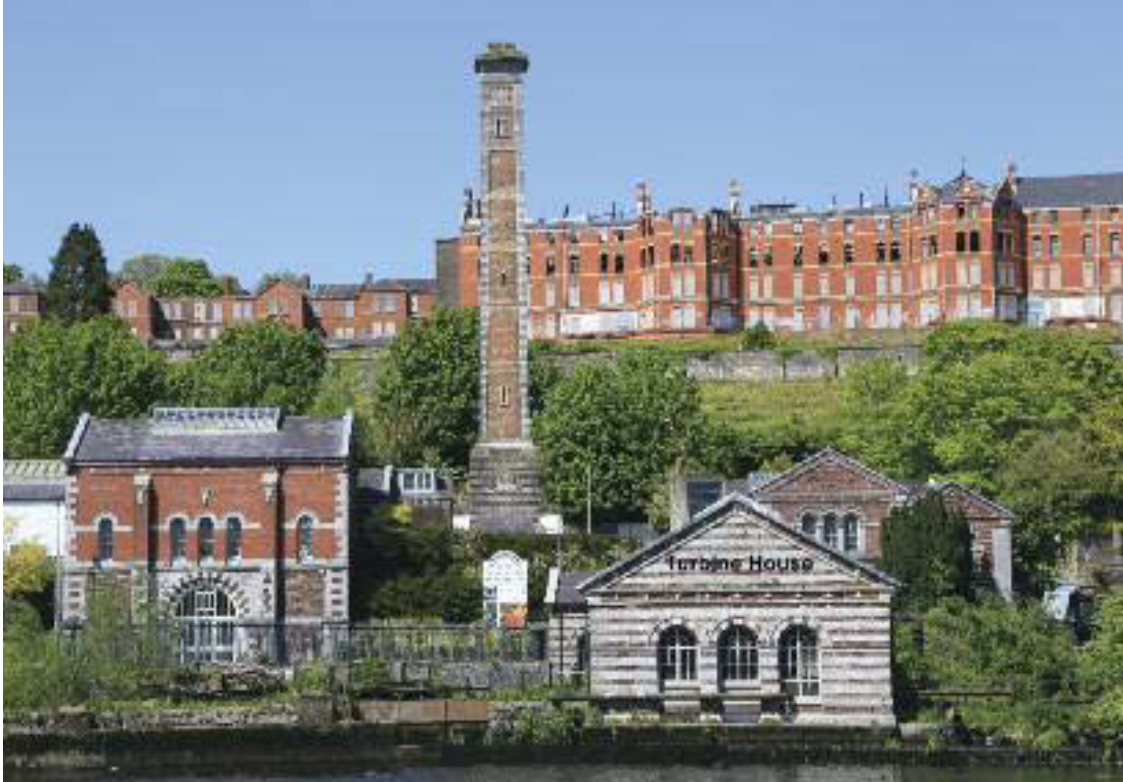
Turbine house of 1888, Cork Corporation Waterworks.
