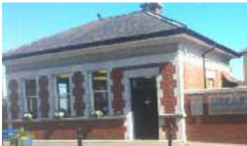
Provincial bank, Schull, built c. 1900, using brick with limestone details.
