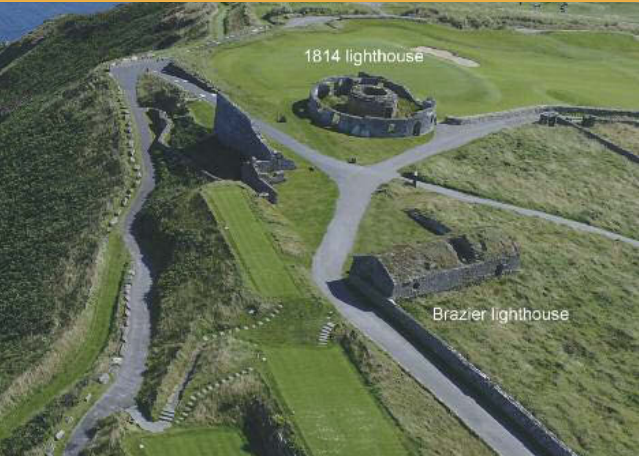
The seventeenth century brazier lighthouse on the Old Head of Kinsale and its replacement of 1814.
