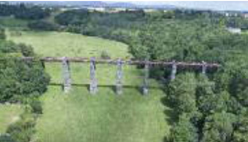
ABOVE: The Kilcummer Viaduct of 1860, on the Mallow to Waterford and Rosslare Harbour line.
