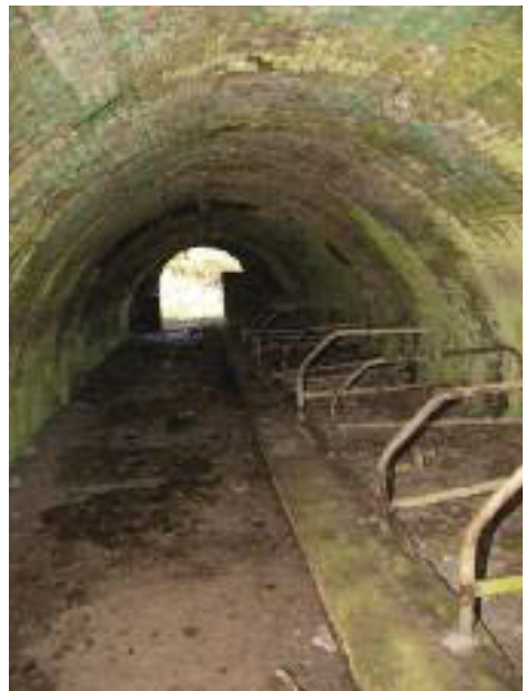
Interior drying chamber in the Hoffmann kiln.
