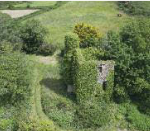
ABOVE: The Cornish Engine house at Glandore manganese mines.
