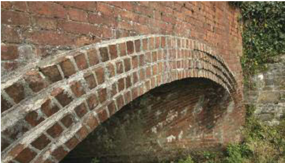
A skewed arched bridge in Bandon.
