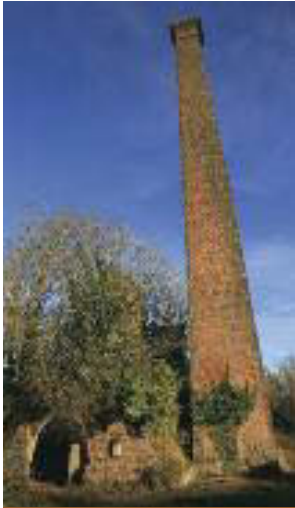
Hoffman kiln of 1895 and stack, at the Youghal Brickwork Company's works at Muckridge near Youghal.
