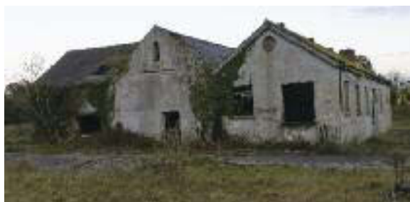
Dromtariffe Creamery showing the west elevation with raised door where milk was delivered into the creamery. Image courtesy of Carol Stack.
