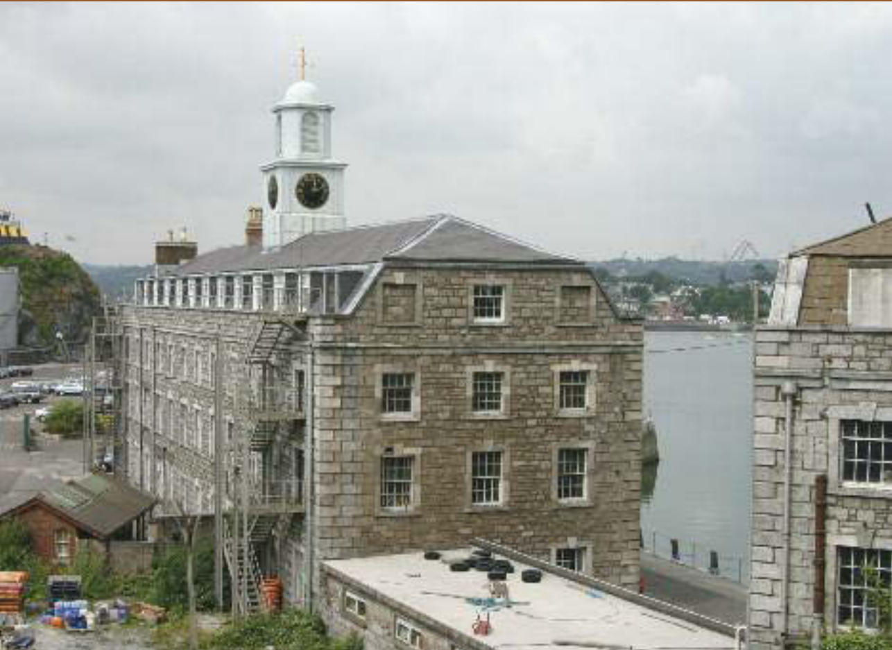
The central storehouse of the northern section of the former British Navy warehouses on Haulbowline Island c.1818, with campanile.
