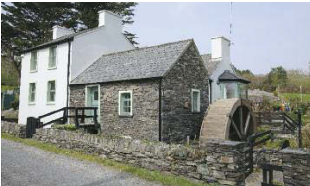
General view of the mill, showing the waterwheel, millhouse and miller's dwelling.
