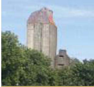
Tall twentieth century silos adjacent to the Shannon Vale Mill (John Phair).
