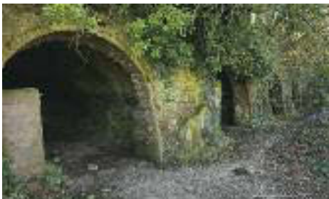
Drying chambers, Youghal Brickwork Company's Hoffmann kiln.
