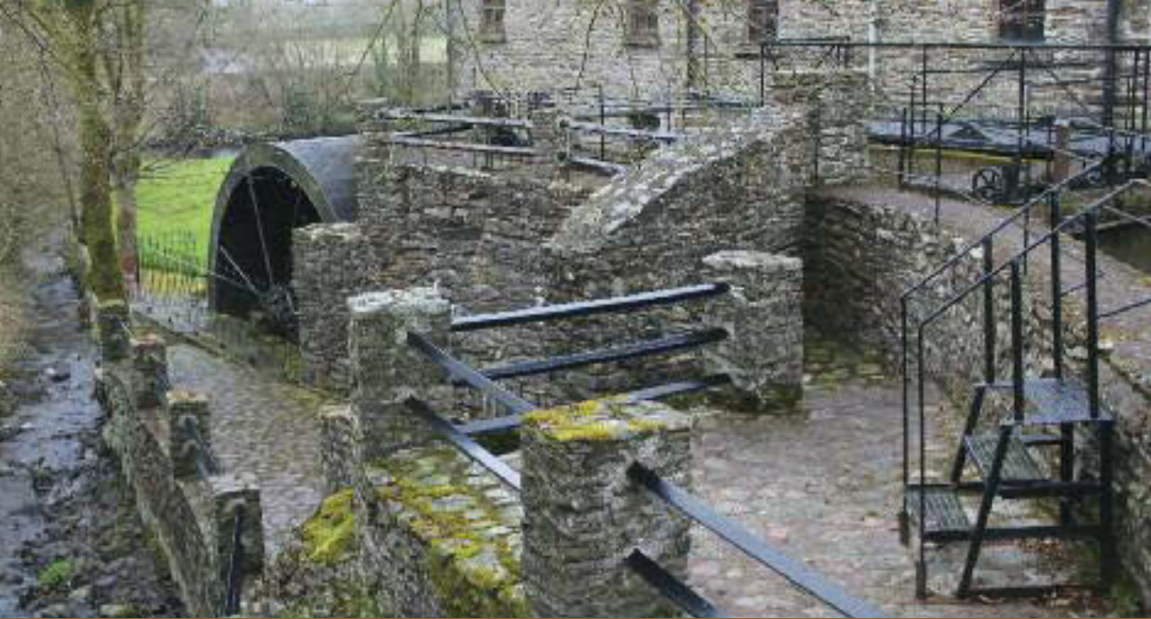
Bealick Mills, Macroom, showing position of waterwheel relative to mill building. Note the height of the stone aqueduct directing water onto the wheel, and the slope away from the wheel.
