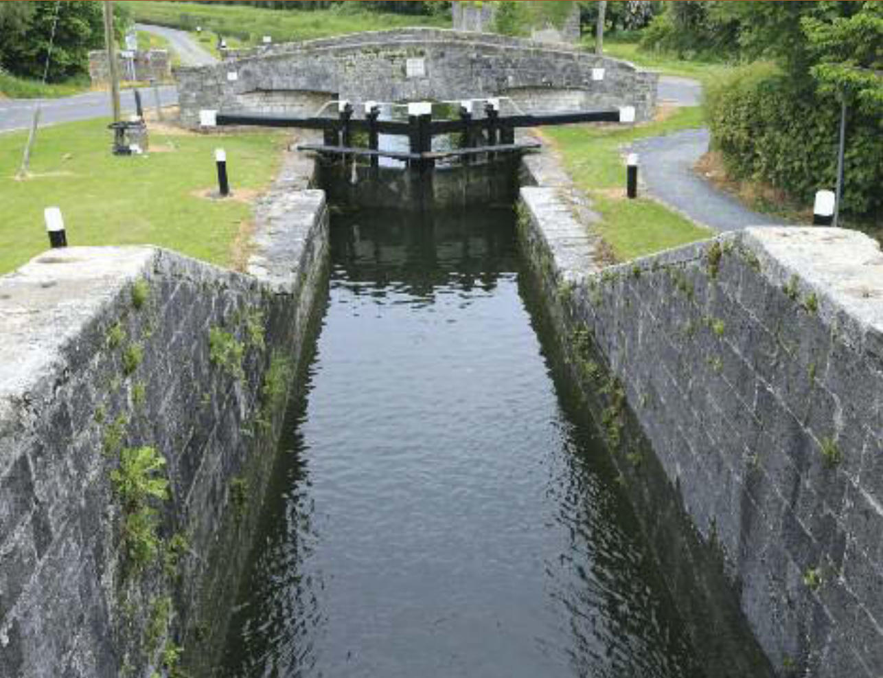
Eighteenth-century lock on Grand Canal, near Rathnangan, county Kildare.
