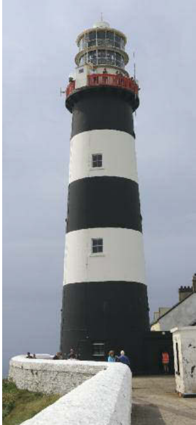
The present Old Head of Kinsale lighthouse, completed in 1853.
