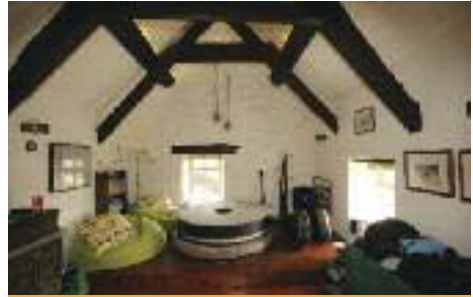
The millstone floor, showing the single set of millstones and the simple collar beam roof truss.
