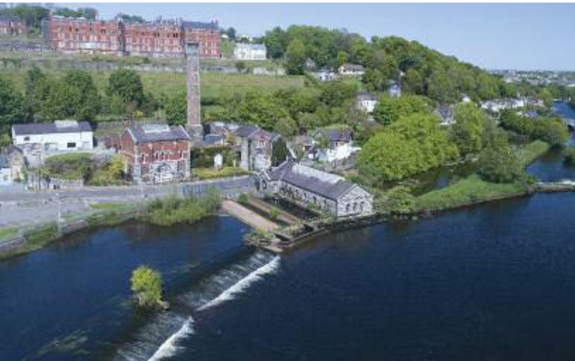
The waterworks weir, Cork. The weir diverts water towards the waterworks and its origins go back to at least the early seventeenth century.
