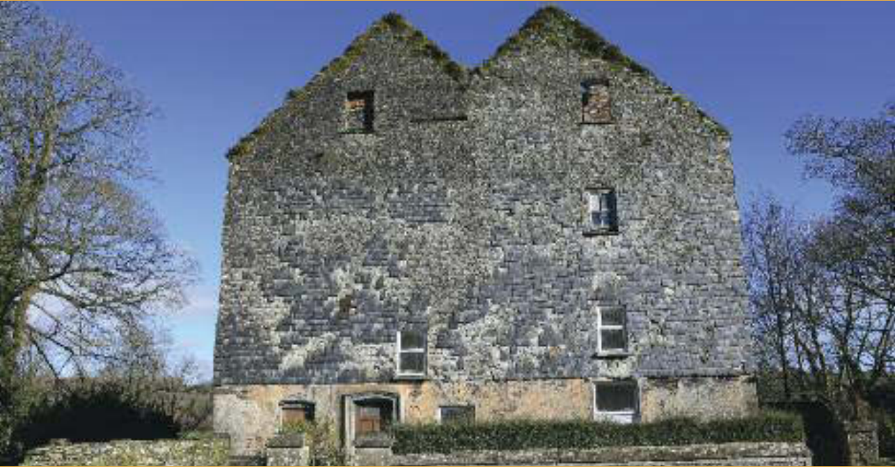
Castleview Mills with its double pile gable end weather slated; door into residential section on the left.
