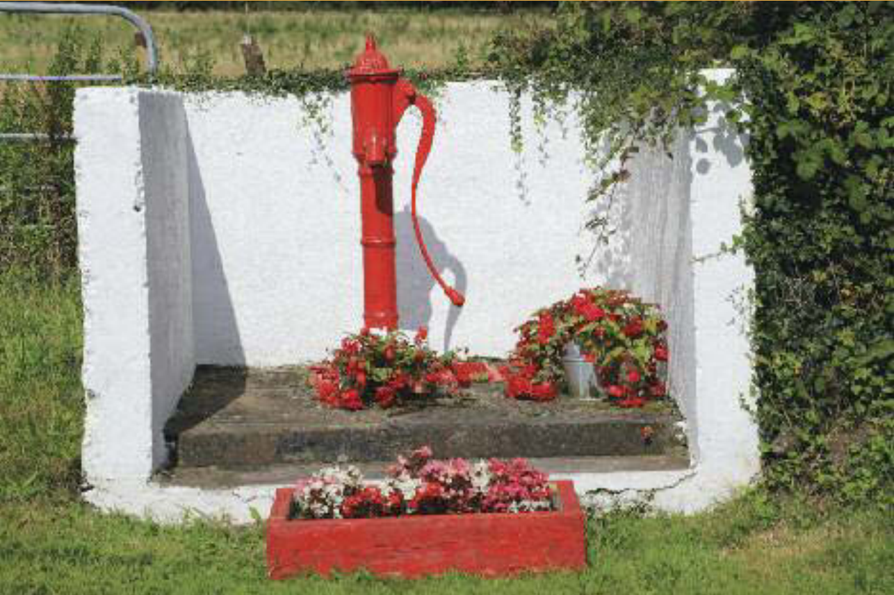
Typical public cast iron water pump provided by County Council with characteristic 'cow's tail' handle, at Ballincurrig.
