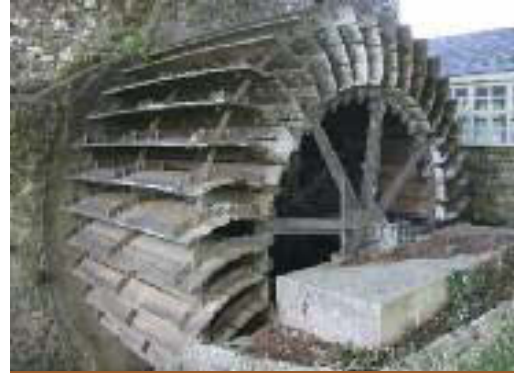
ABOVE: Poncelet type undershot waterwheel at Glanworth Woollen Mills.
