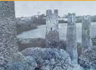
'Leader's Aqueduct' - This aqueduct was built c.1860 by Henry Leader of Clonmoyle House, as a philanthropic irrigation project, providing much needed local employment. It consisted of seventeen pillars carrying water, sourced from the River Dripsey, across the valley from Clonmoyle to Knockanenagark (Henmount). The two highest pillars are 25.6 metres/84 feet in height. Thirteen pillars remain, some in ruinous condition. The aqueduct underwent many modifications, but fell into disuse during the late 19th century, when it became known as 'Leader's Folly'. Text and image provided by Doug Lucey (ACR Heritage).
