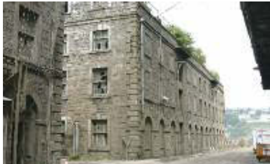
West-facing elevation of former British Navy storehouse on Haulbowline Island, c.1818.
