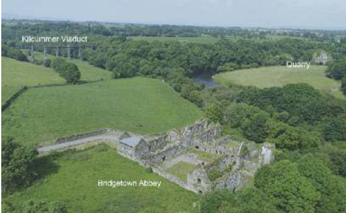
Remains of likely later medieval quarries at Bridgetown Abbey, near Castletownroche, Co. Cork.
