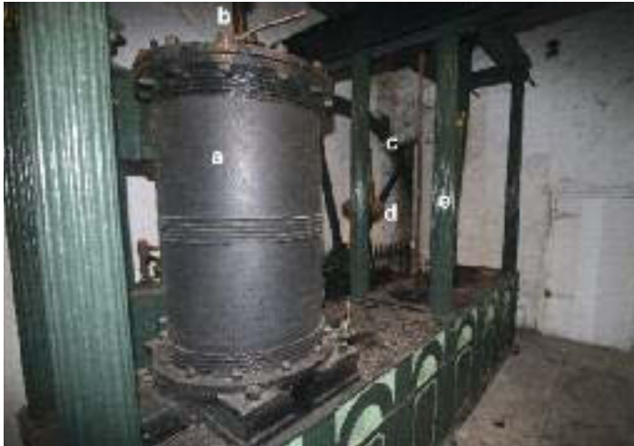
Six-column independent beam engine, in situ, at Midleton distillery: a, piston cylinder; b, piston rod; c, flywheel; d, governor; e, supporting column.
