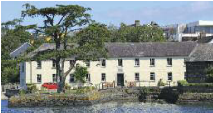
Two-storey fish box factory of c. 1820 at Scilly Point, Kinsale. In the foreground the graving dock with its stepped stone sides can clearly be seen.
