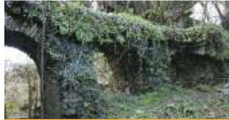
Aqueduct for delivering water to suspension waterwheel at Overton Cotton Mills, c. 1802.
