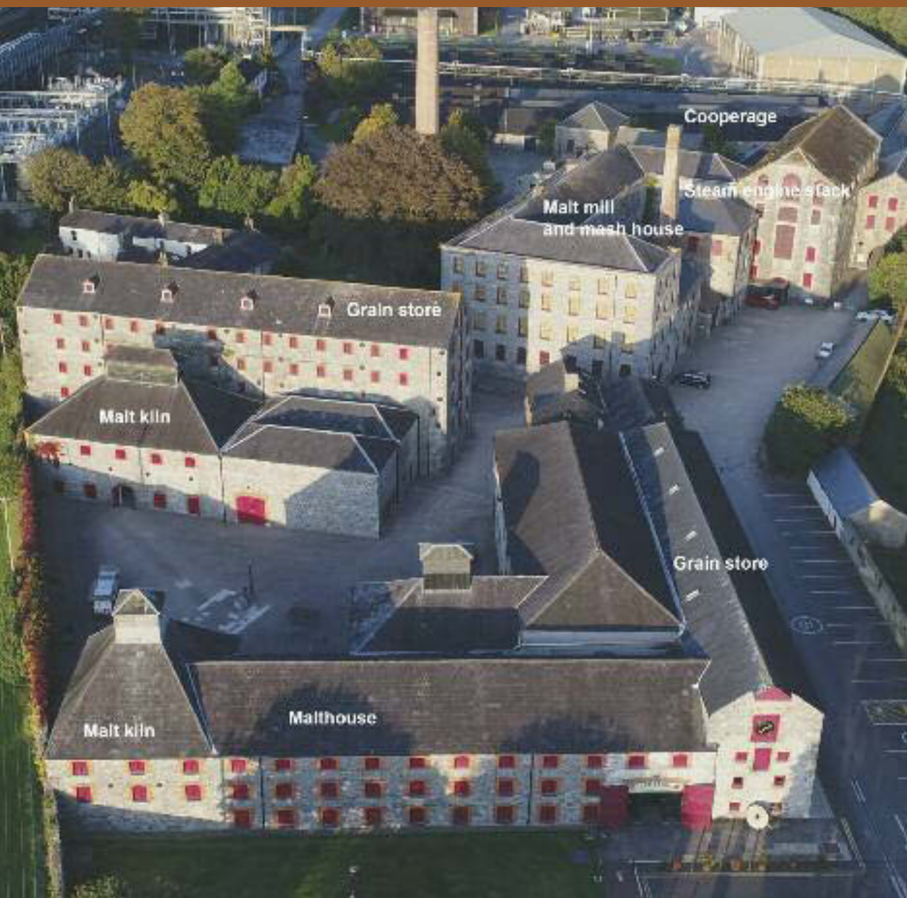
Aerial view of Midleton Distillery showing main buildings. The malt mill and mash house complex is situated within Marcus Lynch's woollen mill of 1793.
