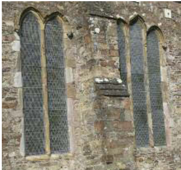
Yellow Dundry stone used in window dressings at St Mary's Collegiate Church, Youghal.
