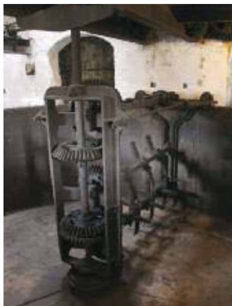
Inside late nineteenth century mash tun at Kilbeggan Distillery, county Westmeath, showing rotating arms and the copper plates at the base, designed to retain heat.
