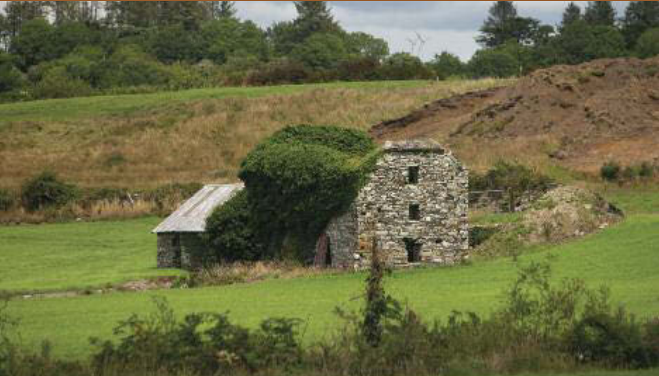
The Tuck and Corn mill at Inchinagotagh. The two-storey building in the foreground is the Corn mill; the single storey Tuck mill is in the background. The mill race ran in between.
