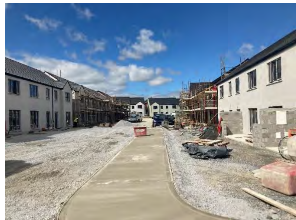
Units under construction in Carrigaline
