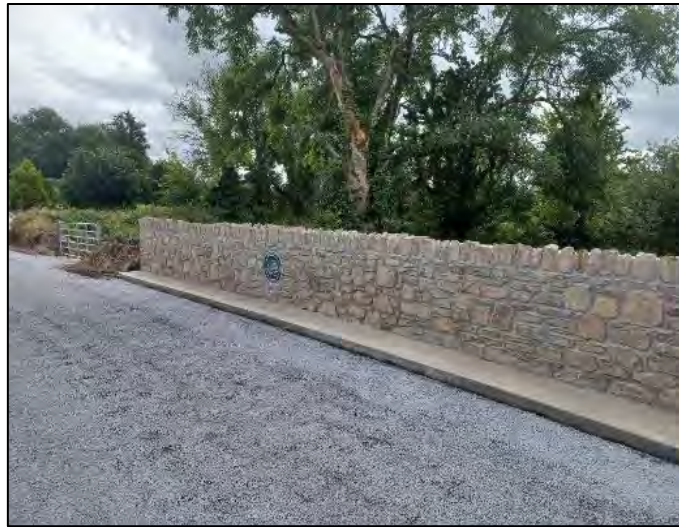
Replacement of L6027 Maulnarouga North Bridge
