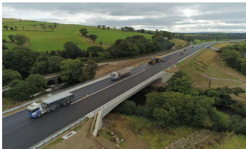
N22 Baile Bhuirne Macroom Road Development – River Lantry Bridge.
