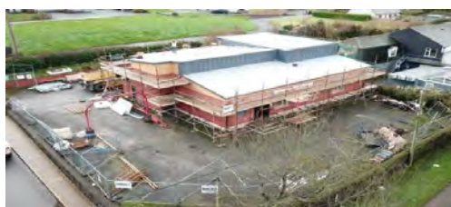
Ringaskiddy Community Centre Roof Repair
