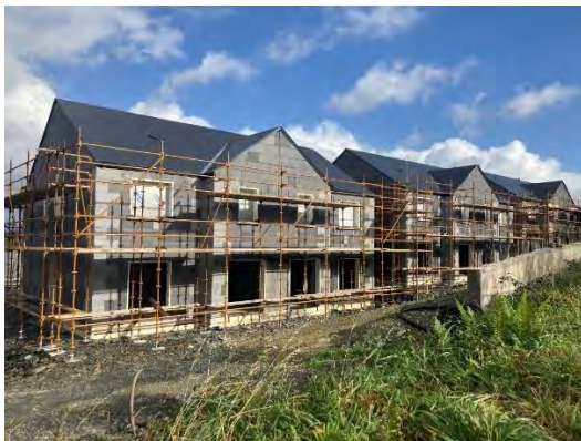
Units under construction in Bantry
