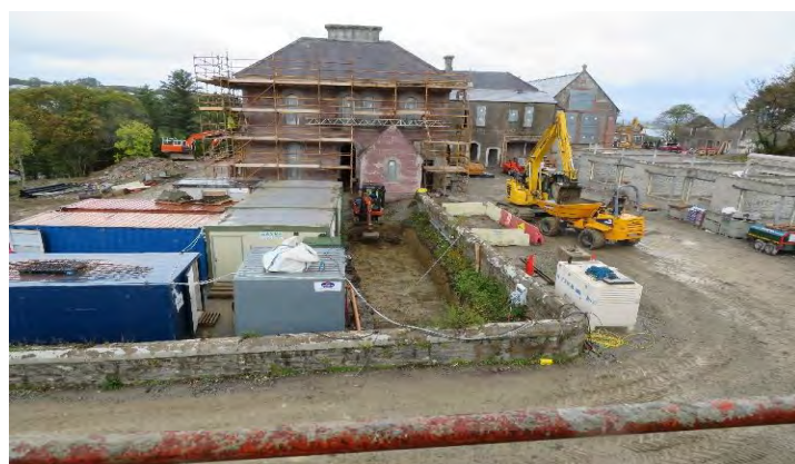
The construction of 18 units commenced in the former Bantry convent
