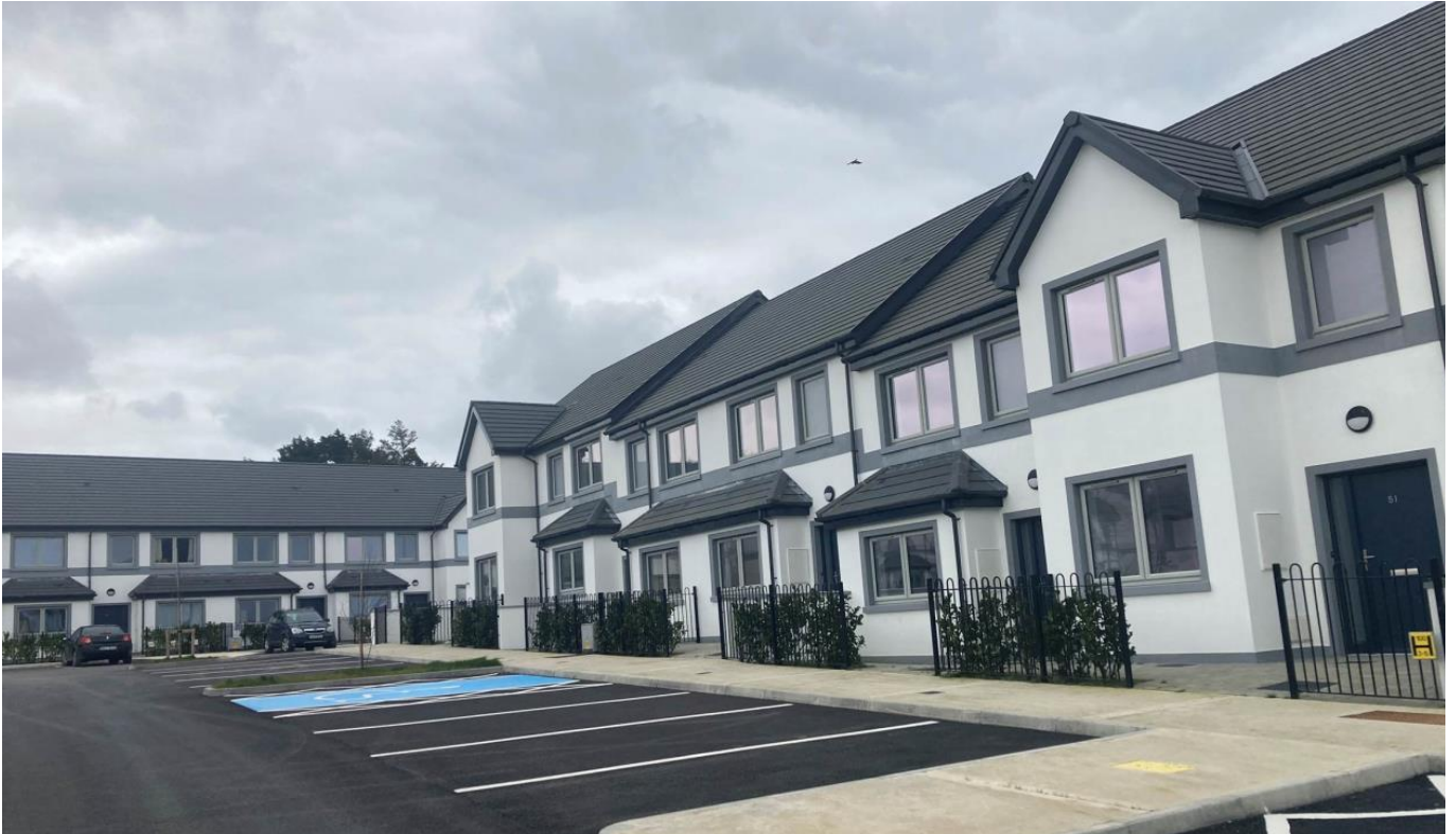
Completed Social units in Kinsale
