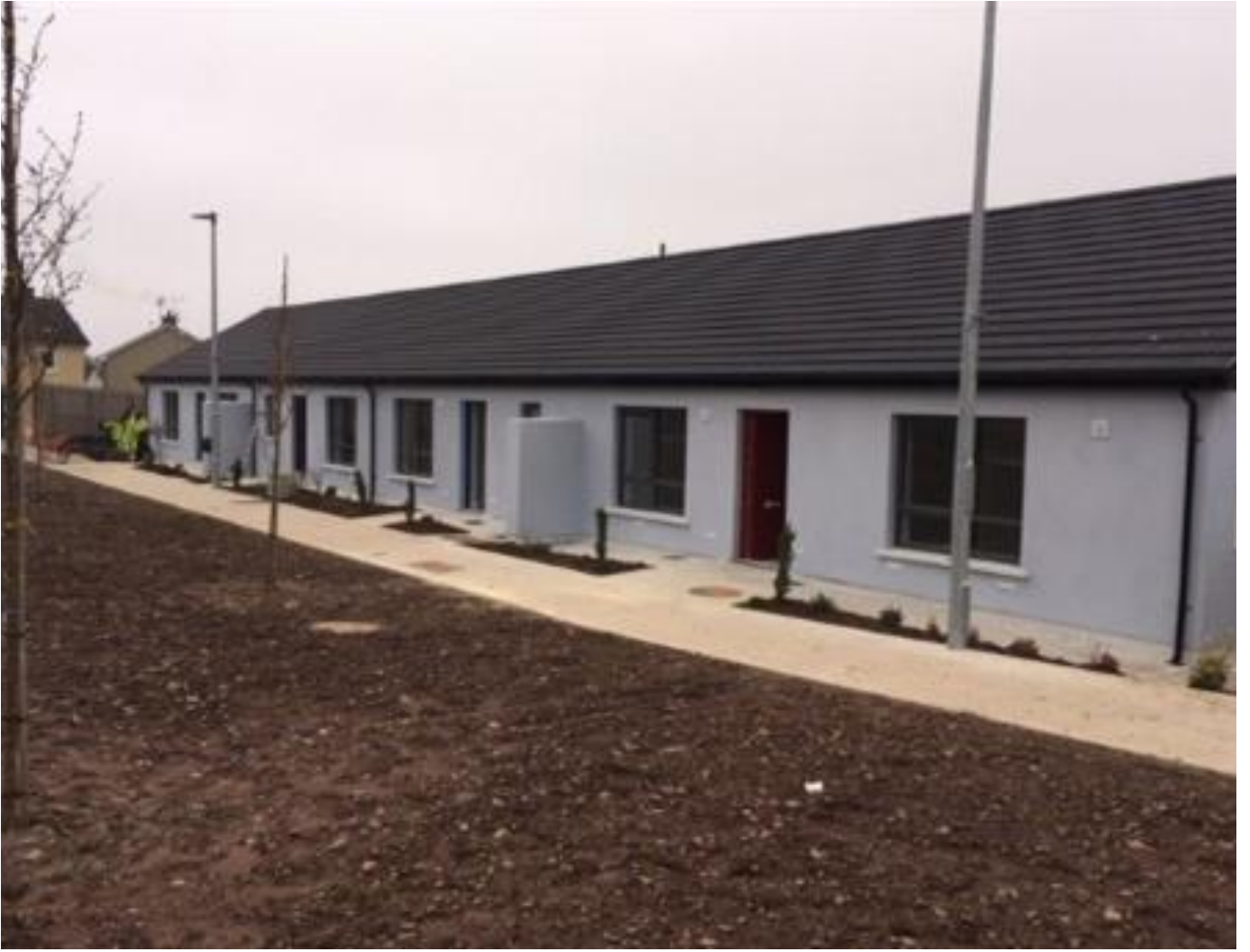
Completed OPD Design & Build units Mallow
