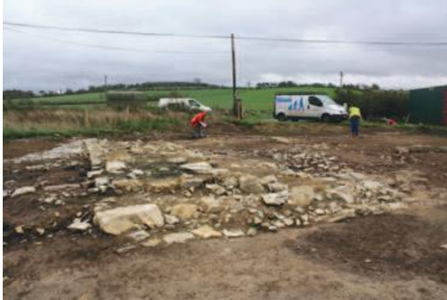
Foundations of Caherduggan Castle as revealed by archaeological excavation. Image courtesy of Rubicon Heritage.
