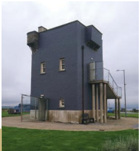
Exterior of the old Signal Tower, Old Head of Kinsale.
