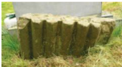
A moulded jamb section reused as a headstone.
