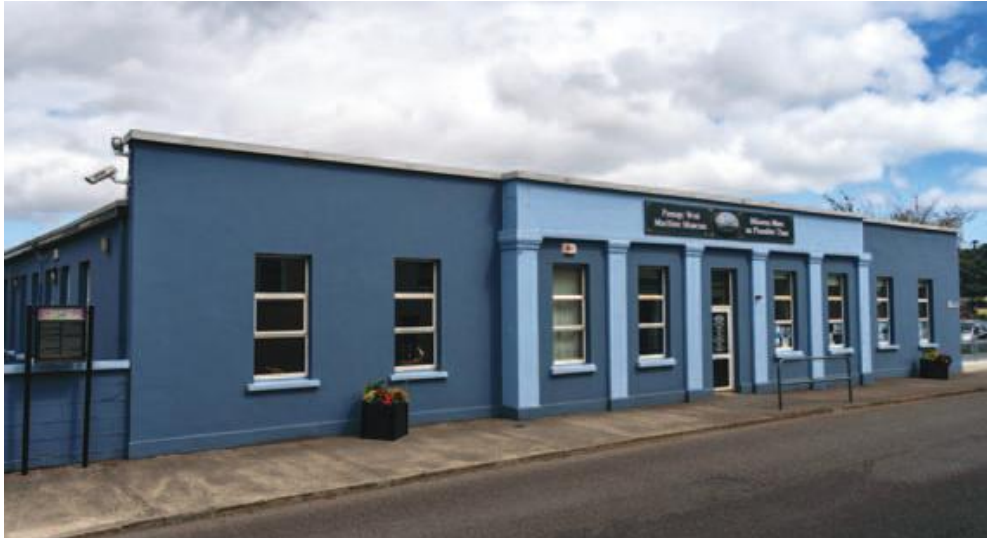
The exterior of Passage West Maritime Museum.
