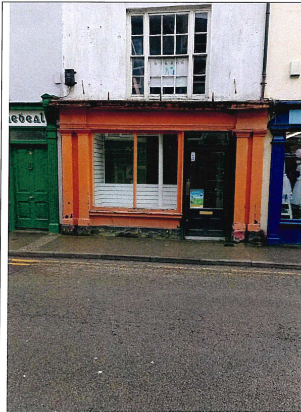
Existing Front of No. 42 North Street
