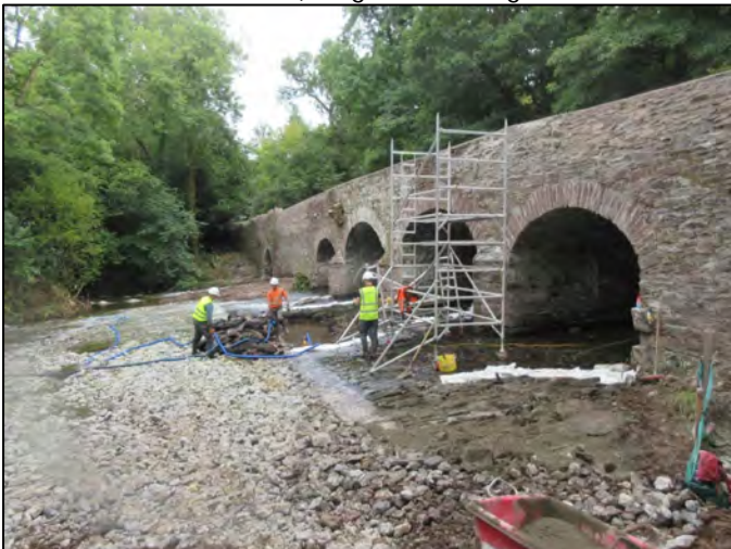
Refurbishment of L2205 Rycourt Bridge
