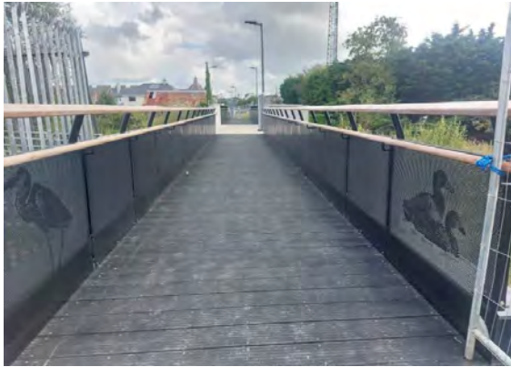
Lodge Park Bridge Midleton
