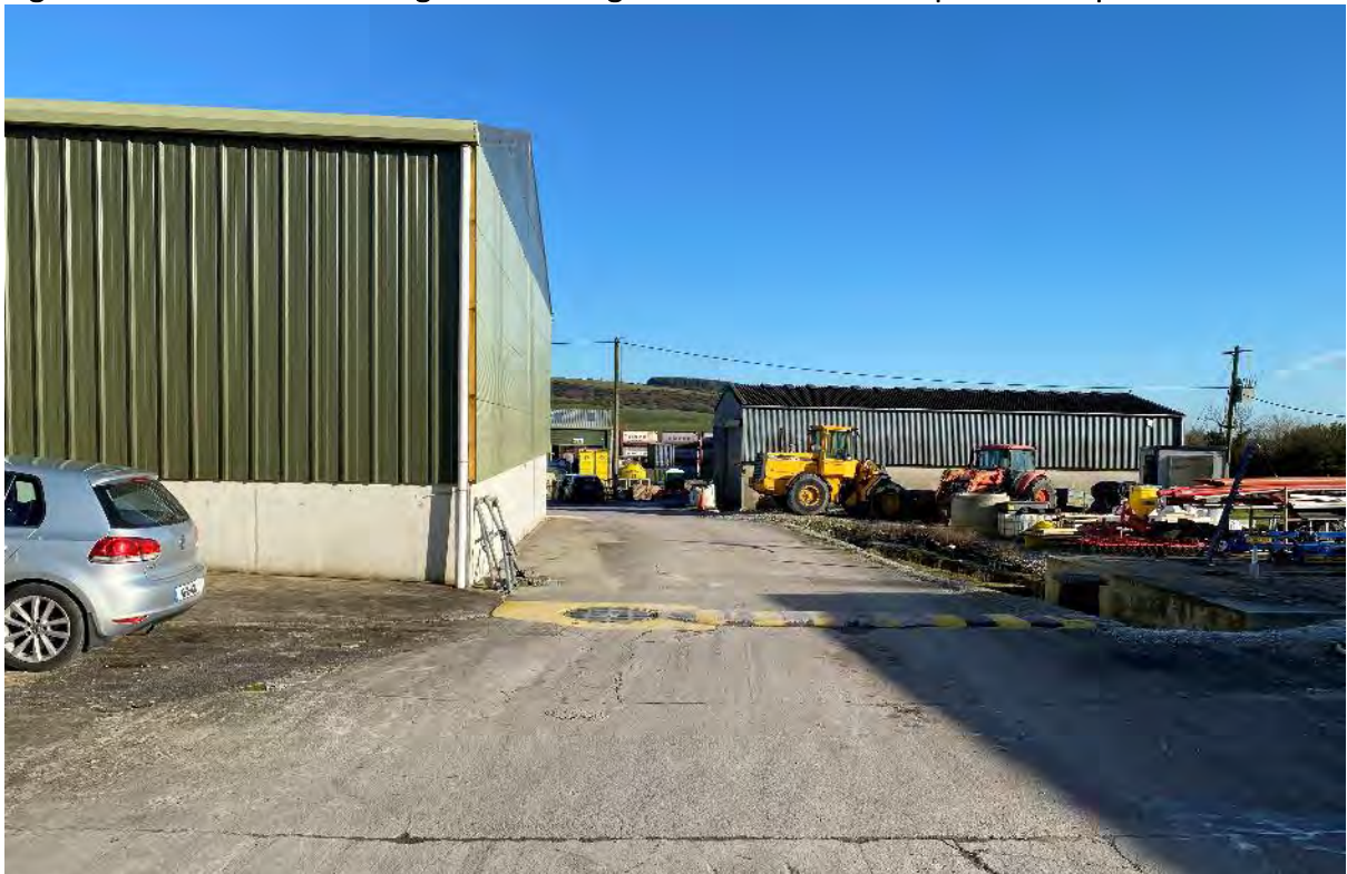
Figure 4: Access Route through the Existing Yard towards the Proposed Compound
