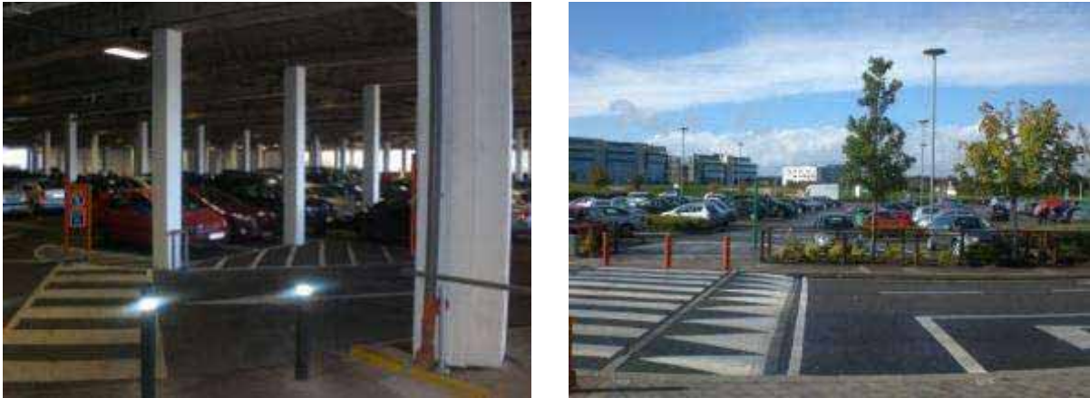
Fig. A5.3.4, A5.3.5: Surface and undercroft (below Tesco) car parking
