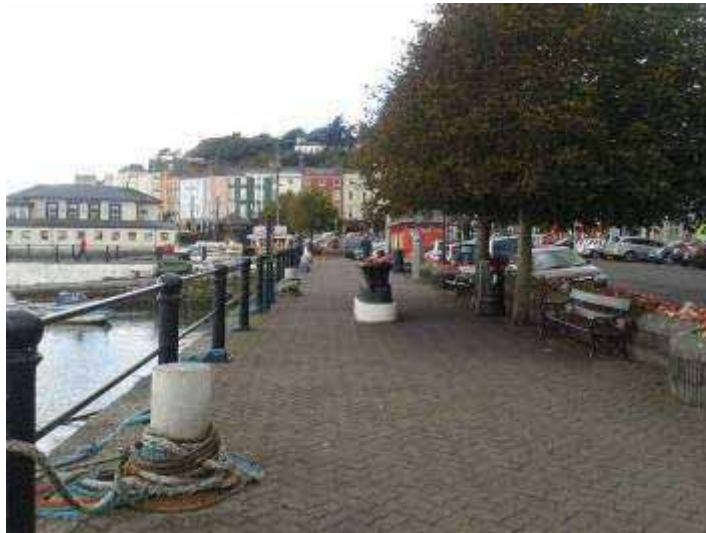
Fig. A5.6.9: Harbourside Promenade: Public realm in need of upgrading
