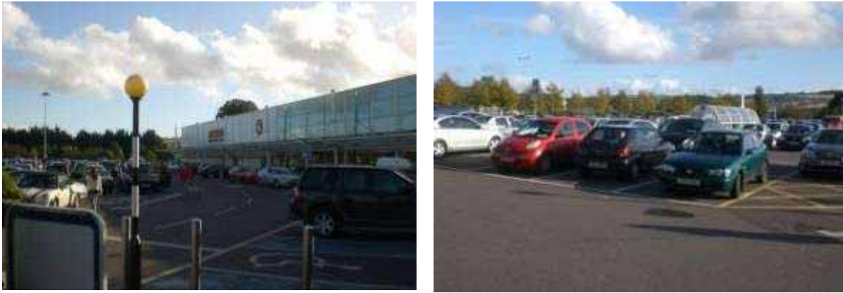
Fig. A5.3.14, A5.3.15: Poor quality urban environment dominated by surface car parking
