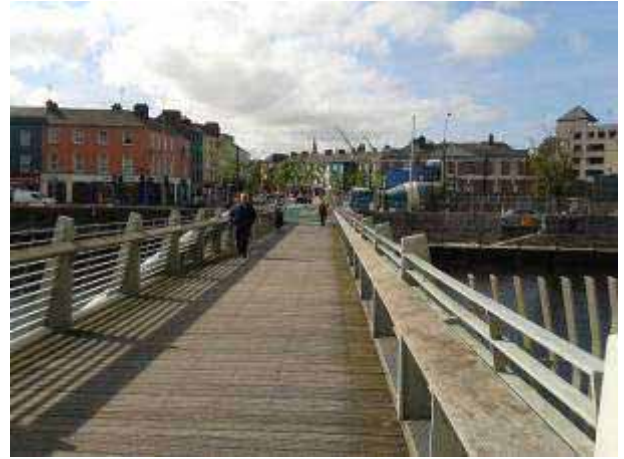
Fig A5.2.13: Pedestrian Shandon Bridge
