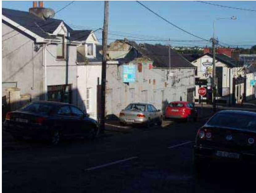
Fig. A4.9.4: Derelict site at the junction of Church Hill/Kilmoney Road
