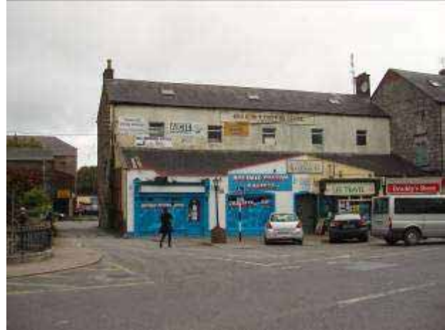
Fig. A4.8.5: View of site from Main Street
