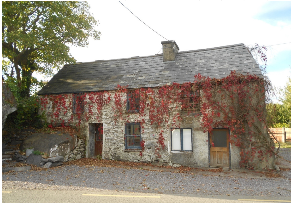
Figure 2.11 Vernacular building in Cúil Aodha built incorporating a rocky outcrop
