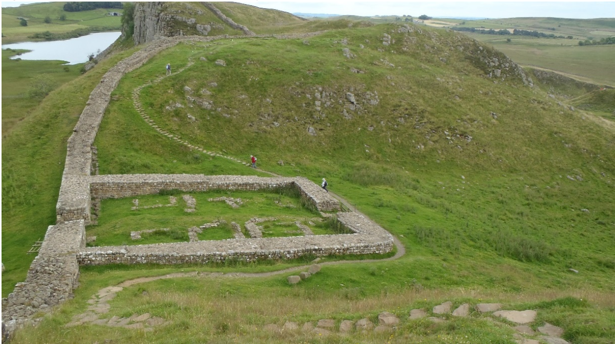
Figure 10.35 Natural stone steps, Hadrian's Wall, UK
