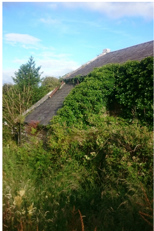
Vegetation growth throughout the bell tower and on north side of roof
