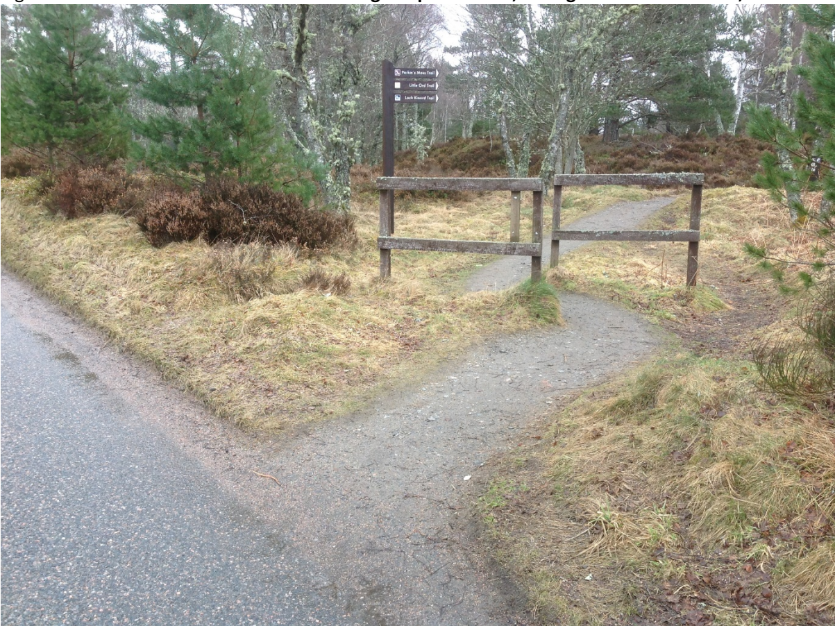
Figure 10.36 Timber barrier at edge of public road, Cairngorms National Park, UK
