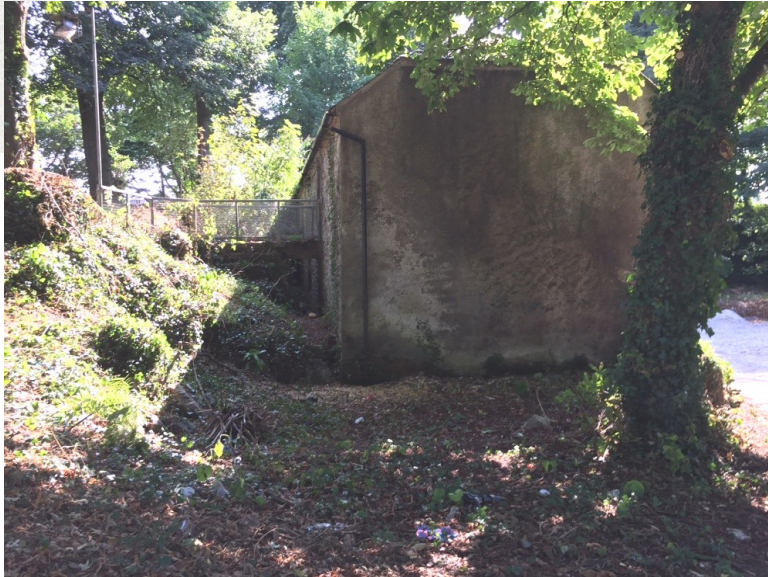
Embankments for wild pollinator nesting at Midleton Lodge Park & Midleton Northern Relief Road
