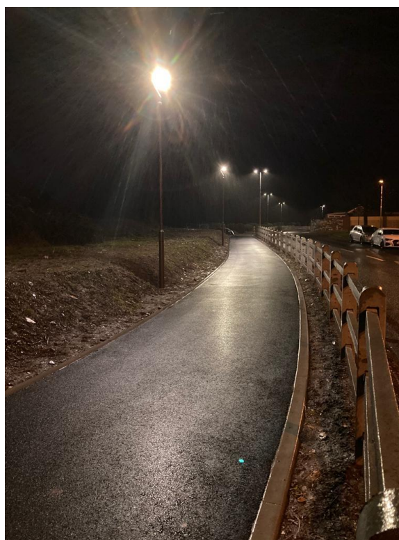
Typical cycleway lighting
