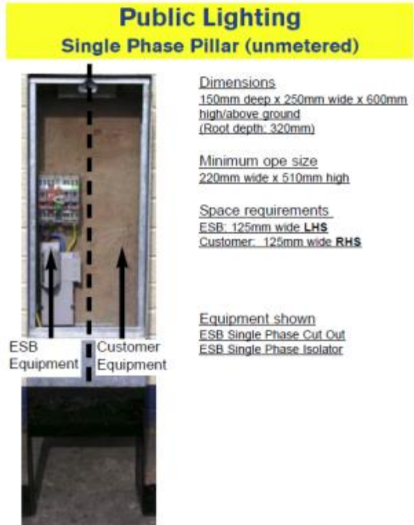
Figure 8: Unmetered/Metered Lighting Pillar with ESB equipment
