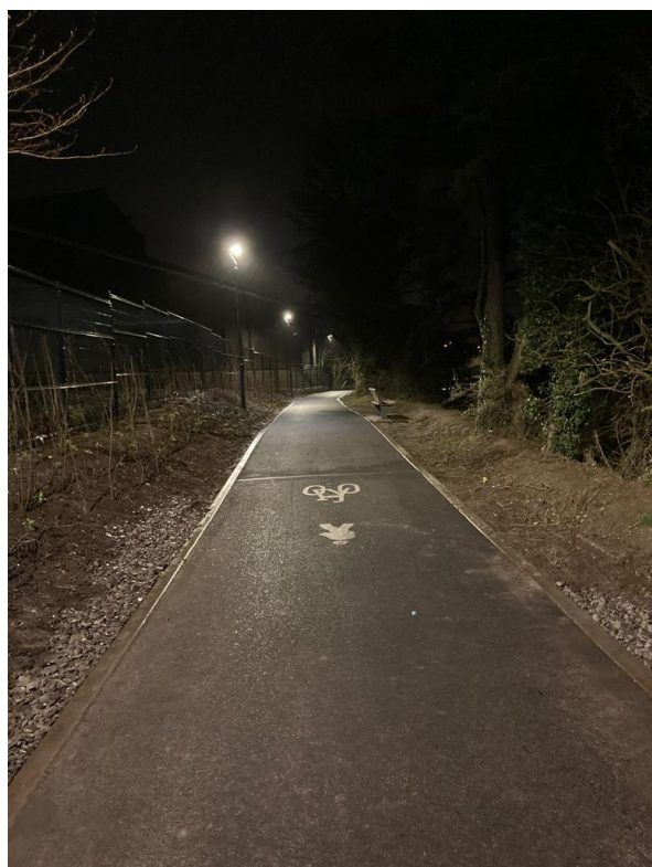
Typical walkway lighting
