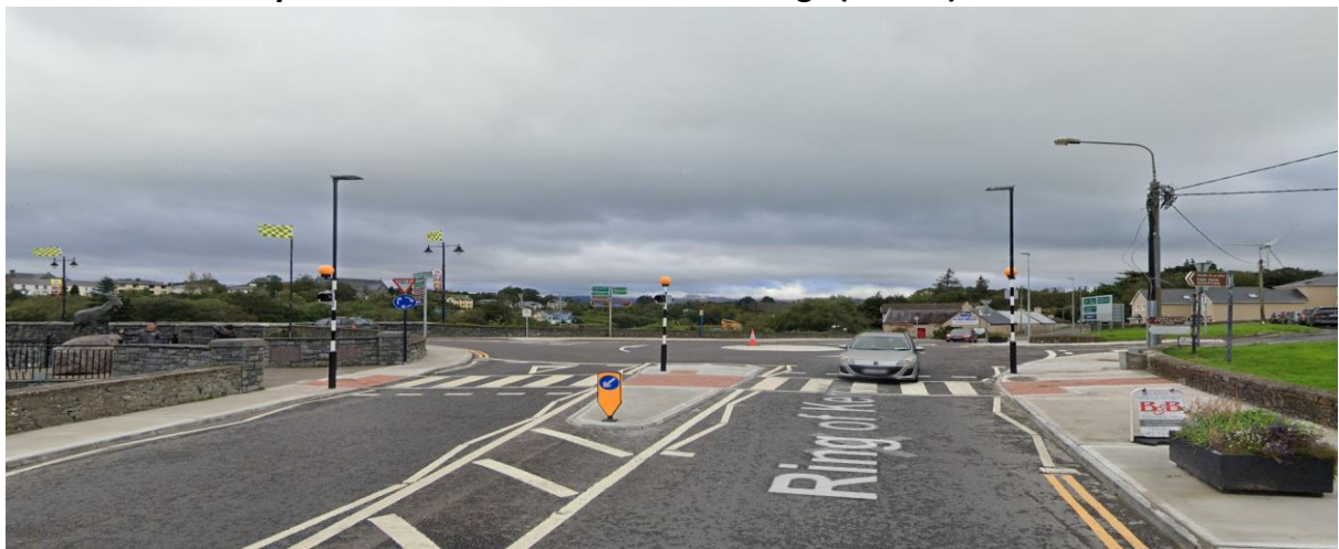
Zebra auxiliary lighting integrated into traffic signals
