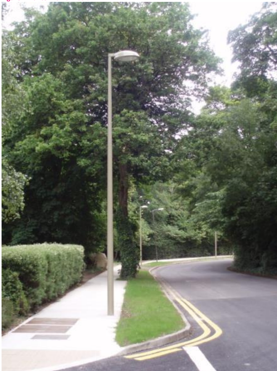
Figure 1: Lantern on 6m Column
