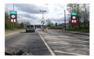
Gateway lighting using supplementary LED lighting on double-headed column in central island. These should be hinged and socketed to allow the column to be lowered for Abnormal Loads
