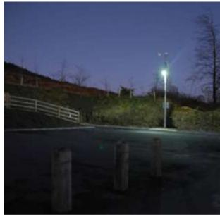
In the Northern Hemisphere it is challenging during winter daylight hours to sufficiently charge batteries so that they will be capable of powering lights from dusk to dawn (16.5 hours approx on 21st December).
