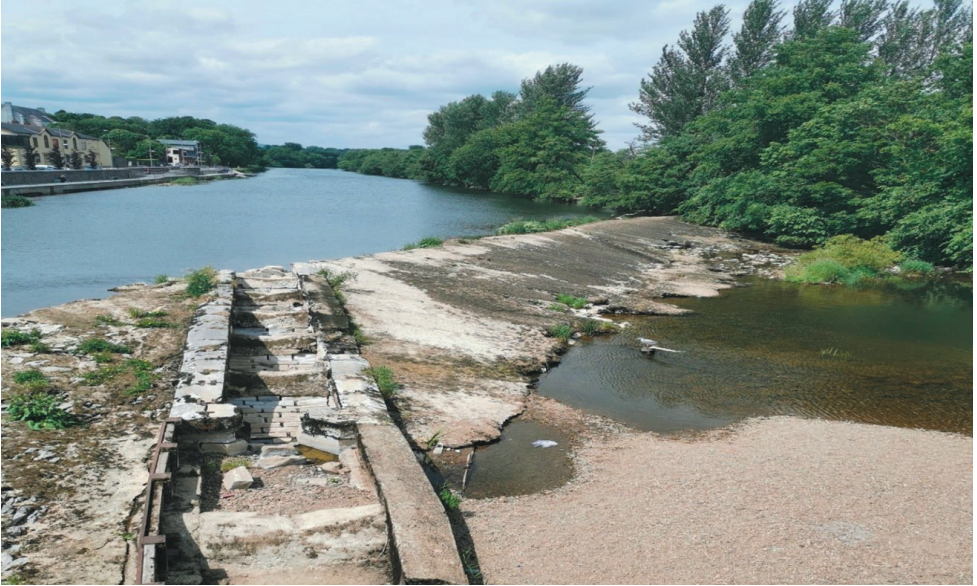
Weir showing dried-out salmon pass. Source: Ger Morrissey
