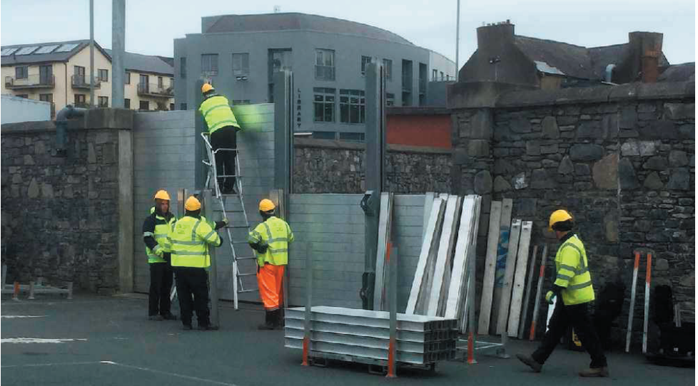
Mallow Flood Defence Wall
