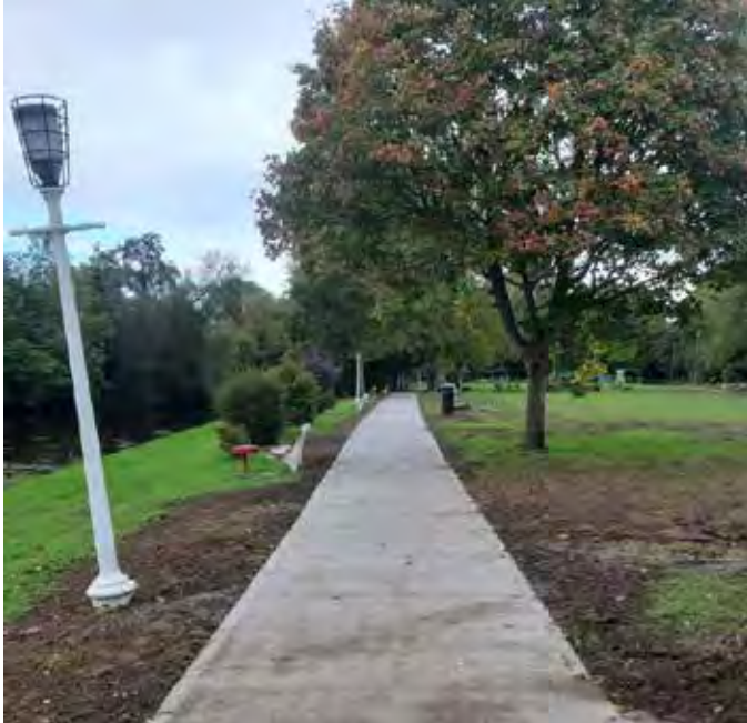
Town Park works completed in Kanturk
