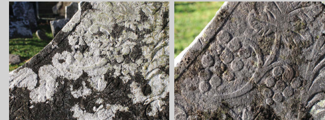
Hand cleaned headstone - before and after
