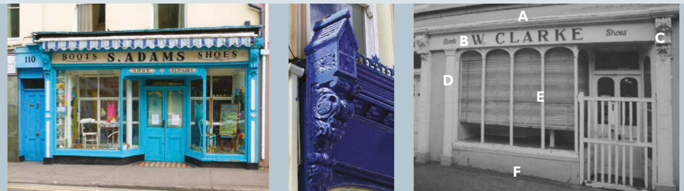
Above: The components of a shop front: A - Cornice, B - Fascia, C - Bracket, D - Pilaster, E - Mullion, F - Stallriser or plinth
