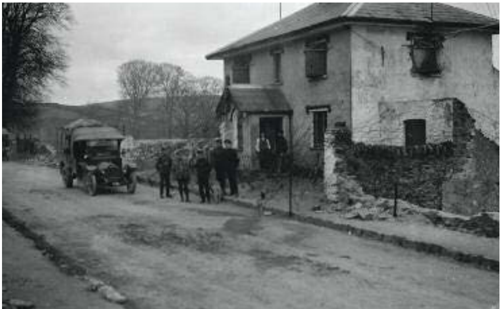
In an effort to defend the RIC barracks, their defences were augmented, particularly with the addition of armour plating over entry points like windows, as can be seen with this example at Ballinhassig.
