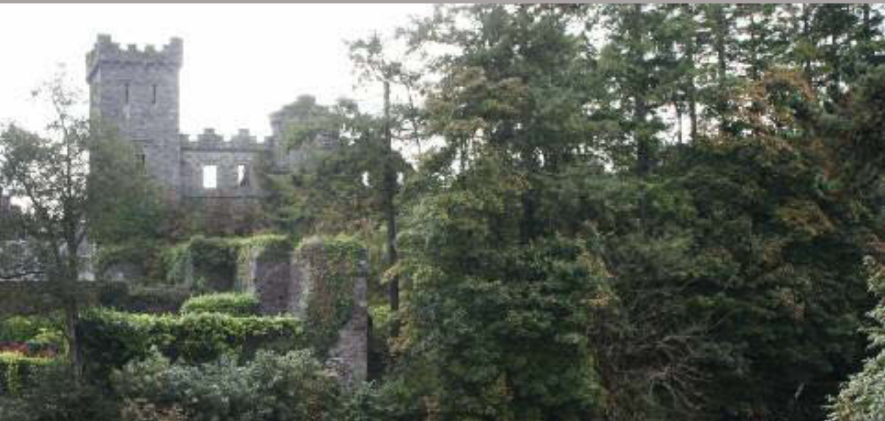
Although Macroom Castle no longer stands, some of the buildings associated with the castle still remain on site.
