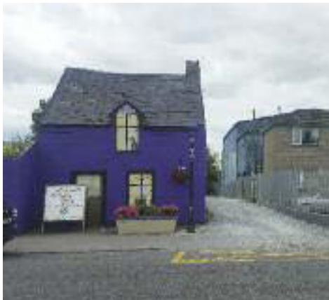
The site of the former Barracks at right, the laneway was a key feature used by the IRA during the attack.
