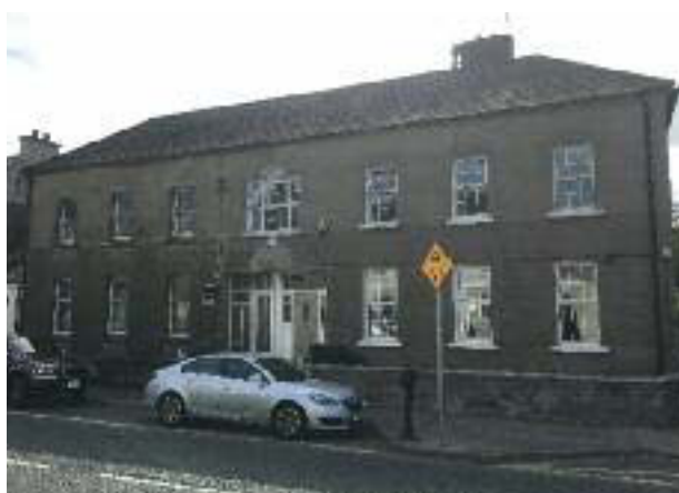
The former barracks in Castlemartyr, outside which Fenian leader Timothy Daly was mortally wounded during the 1867 Rising.
