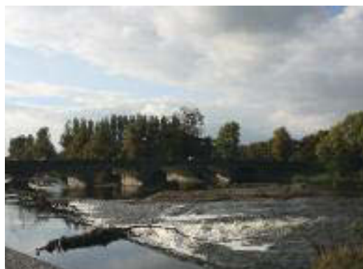
Fermoy Bridge, since May 2016, now known as Kent Bridge.
