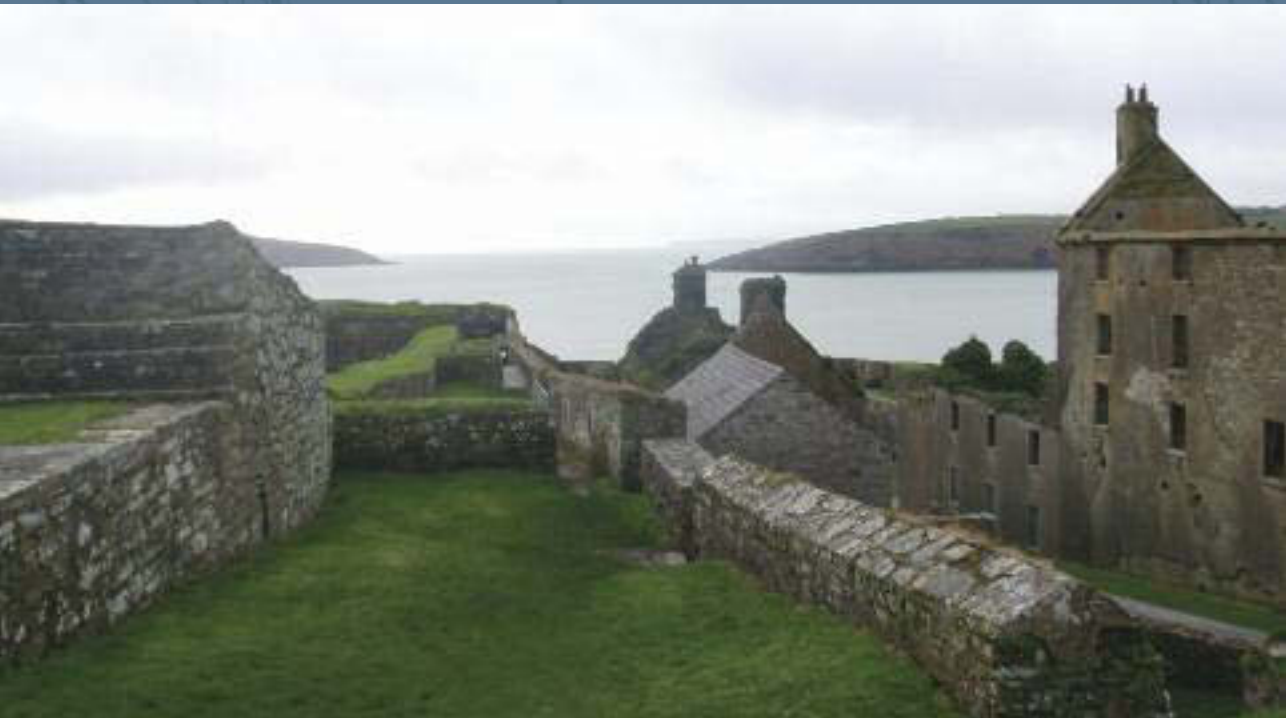
Charles Fort's interior. The buildings were burned in 1922 during the Civil War.
