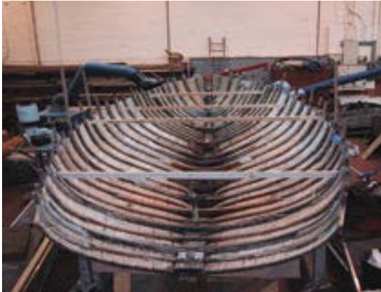
2. The bare hull of the yacht, Fricka , of 1895 after all non-original material was removed. The yacht had been extensively altered during the early 1900's. Her owners, the British National Maritime Museum, wanted her returned to original built form while retaining all existing original material.
