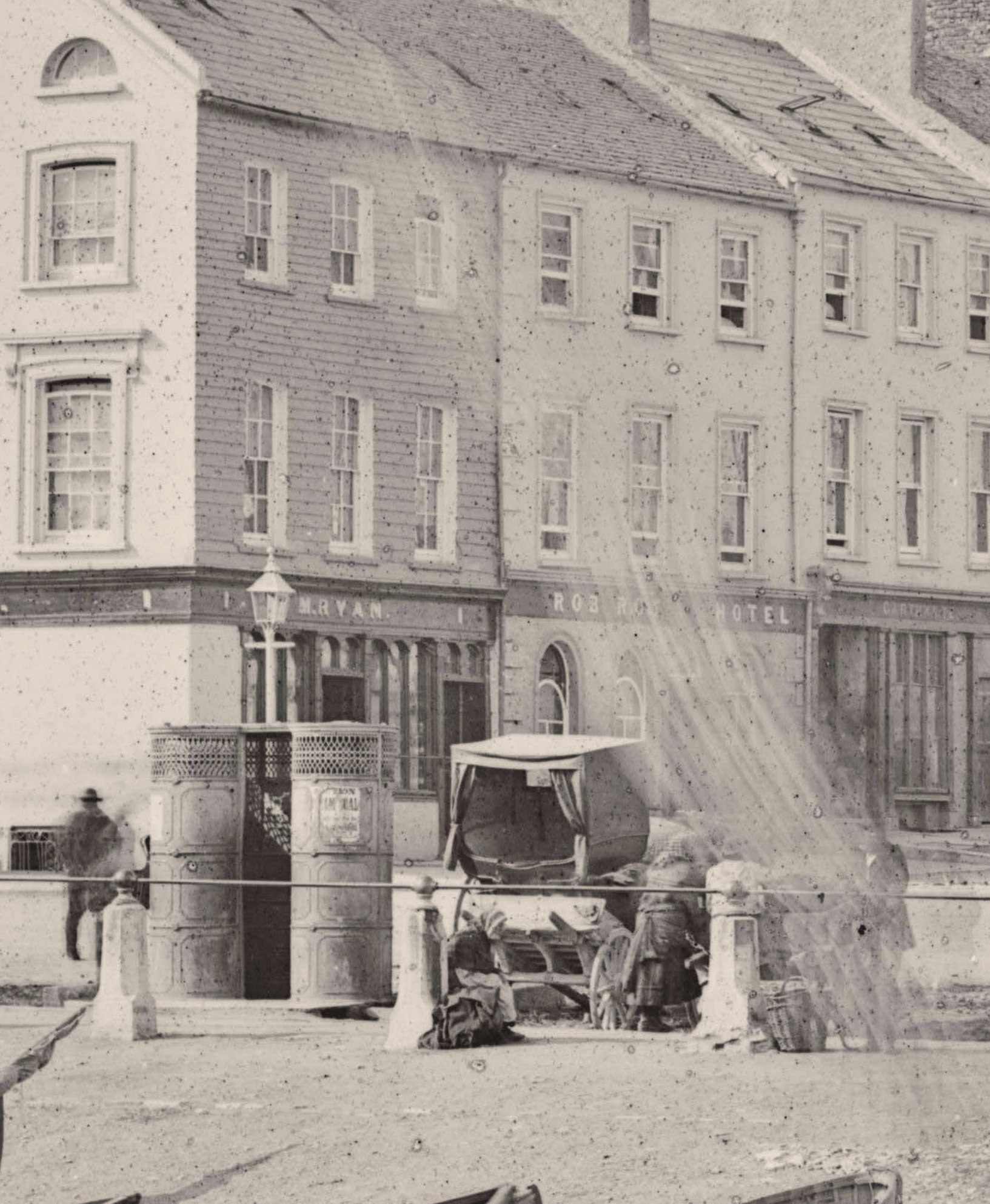
Mid 19th century shopfront with robust glazing mullions and arched top above glazing.
