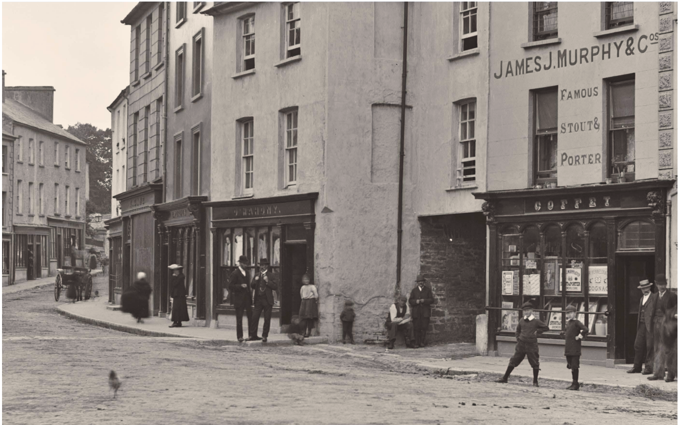
FIGURE 52 BRIDGE PLACE, BANDON Mid 19th century shopfronts with larger glazing and characteristic narrow, tall mullions with intricate column heads to glazing mullions. Note early, tall shopfront without console brackets to left of image. Image from the Lawrence Collection.
