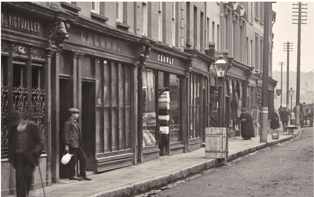
FIGURE 53 SOUTH MAIN STREET, BANDON Early to Mid 19th century shopfronts with large, vertical glazing (replaced to larger, planar glass in the centre shop). Console brackets may have been added in the late 19th century except to the shopfront to the right of the gas lamp. Note the very slender pillasters generally. Image from the Lawrence Collection.
