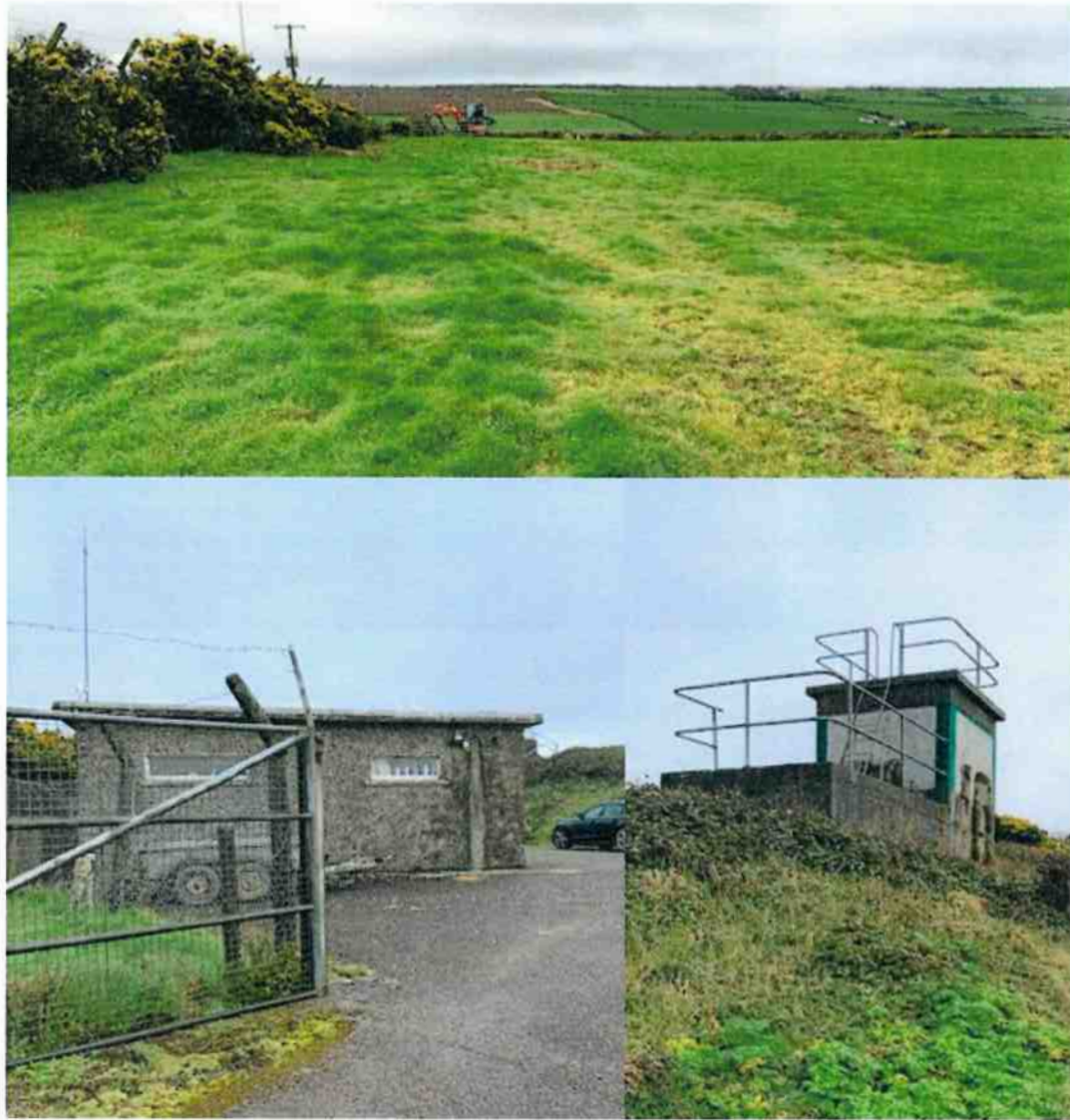
Figure 2 Site Context – Subject Lands (Top) Facing South and Adjacent WTP Infrastructure
