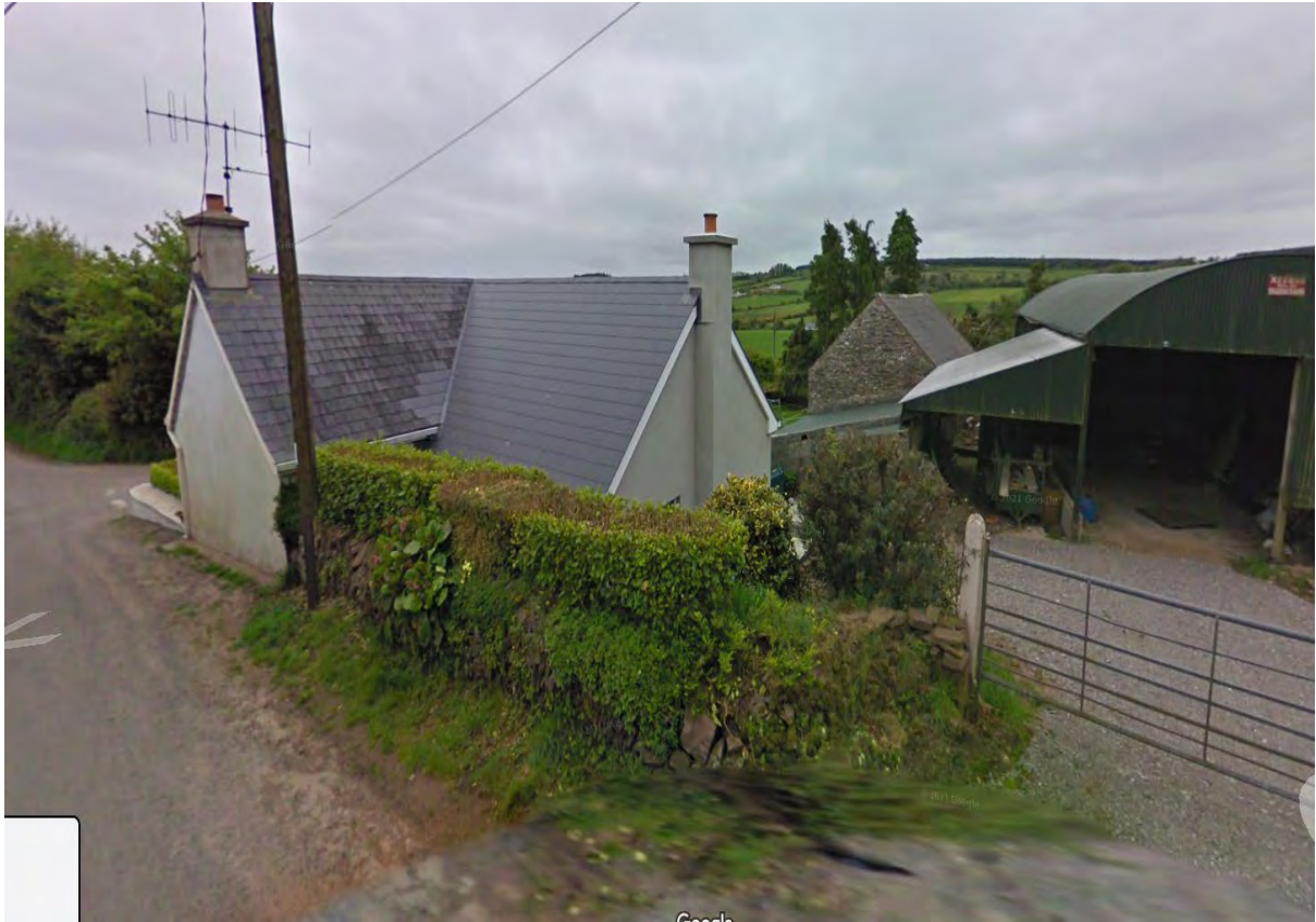
Image showing rear extension subject of this application
