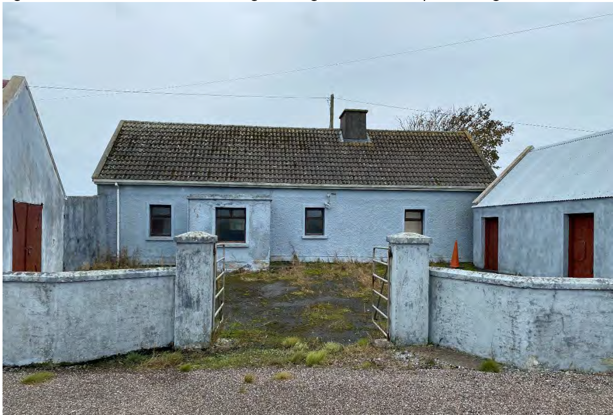
Figure 4: Front Elevation of the Existing Dwelling within its Courtyard Setting
