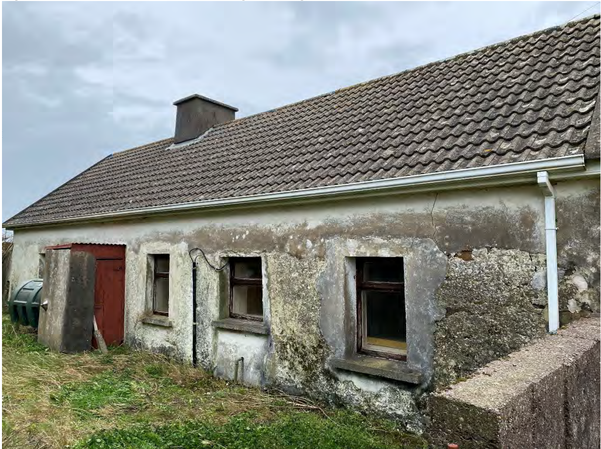
Figure 6: Rear Elevation of the Existing Dwelling
