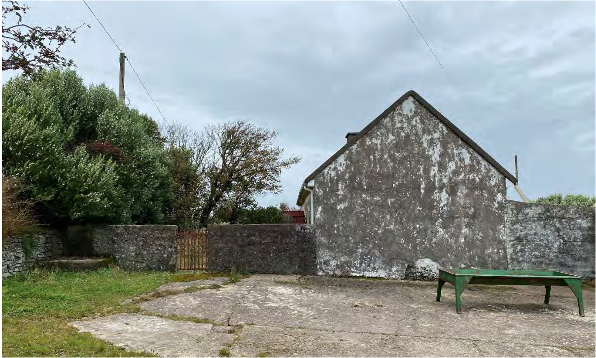
Figure 5: Southern Gable, Side and Rear of the Existing Dwelling
