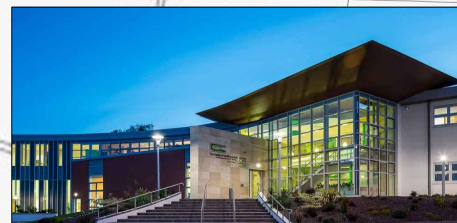
PADDY O'KEEFE CENTRE - EXISTING OFFICE AND ADMINISTRATION BUILDING
