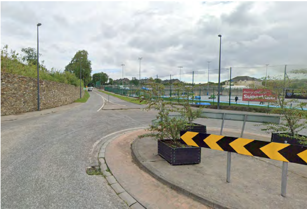
Figure 52 Ballea Road roundabout at Carrigaline United AFC
