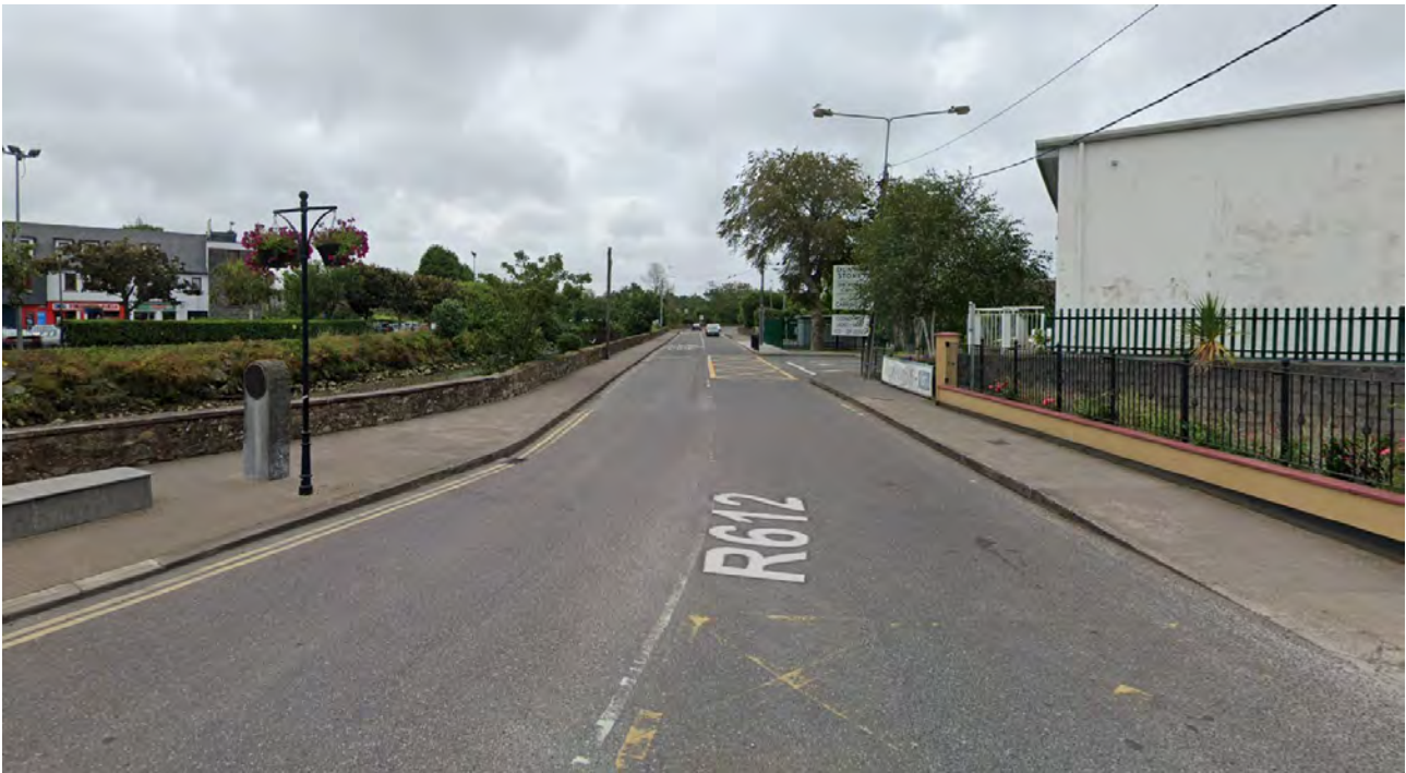
Figure 58 Strand Road western section – Dunnes Stores entrance
