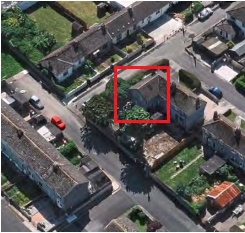
Aerial view of the development
