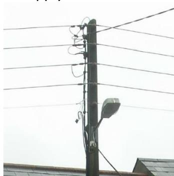
Under Conductor Mounting
