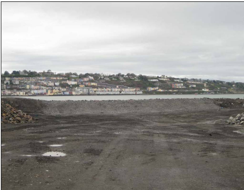
Plate 2 Repair of western sea breach.
