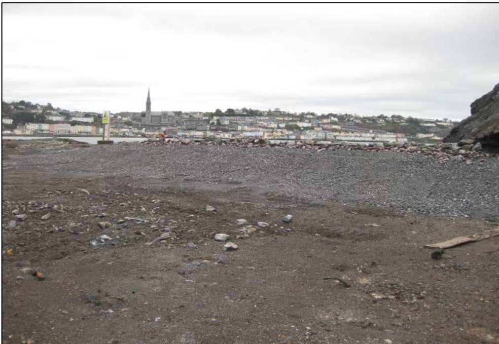
Plate 4 Repair of eastern sea breach.
