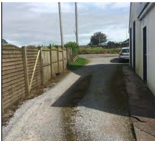
Before Pic - Side View of Rylane Community Centre
