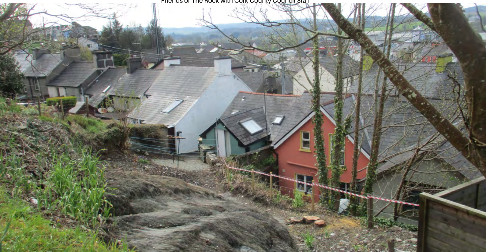
Recently cleared Golden Steps at The Rock to High Street
