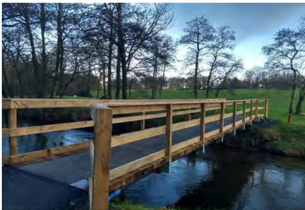
Repairs to Bridge at Mitchelstown Golf Club funded under the 2020 Amenity Scheme
