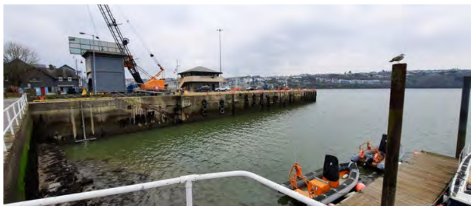
Kinsale Harbour Main Pier
