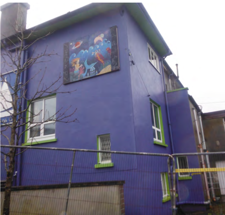
Ballydehob Community Centre Windows
