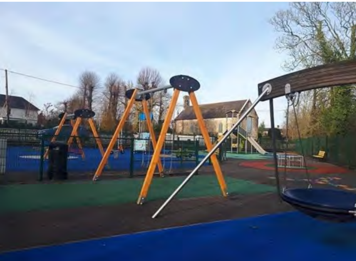
Rathcormac Playground Refurbishment
