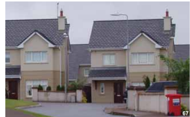
Example of roof types that could accommodate loft conversions
