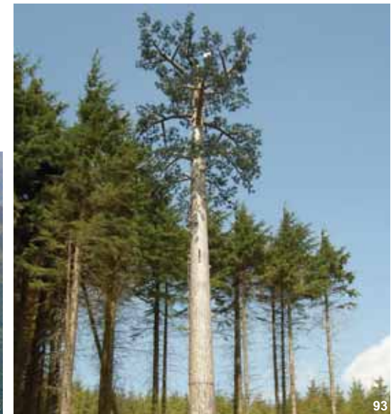
Aerial disguised as a tree
