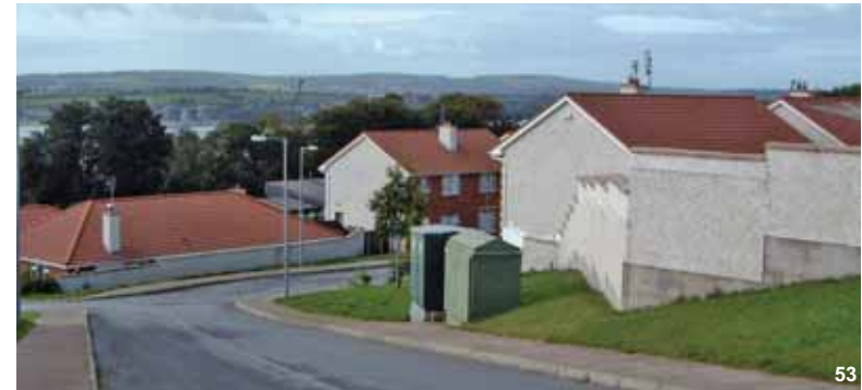
Standard house types unable to accommodate steeply sloping sites without extensive ground works
