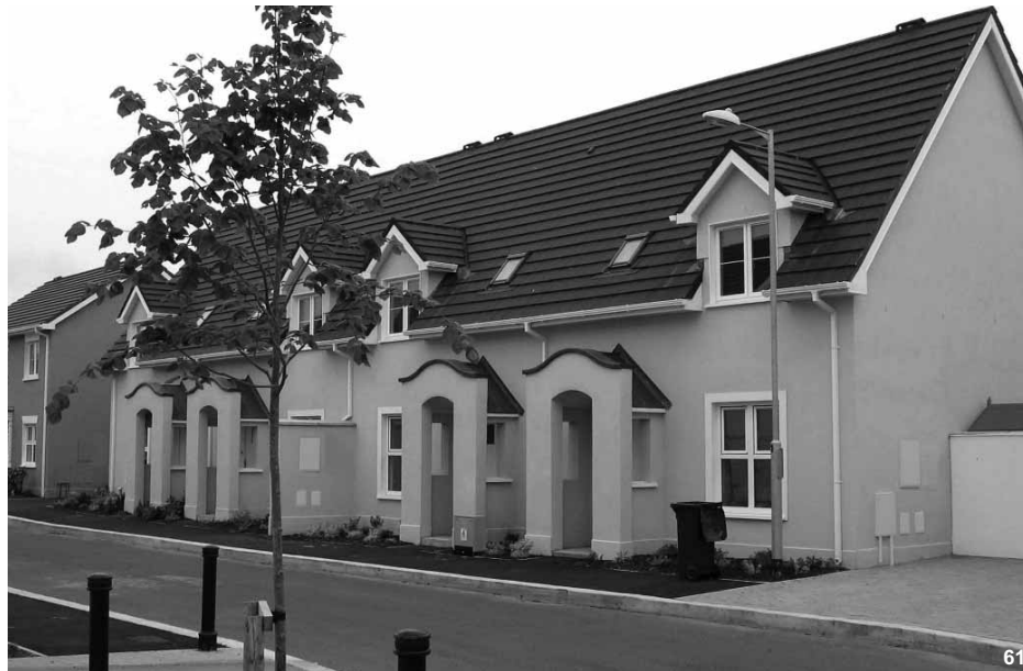
Soil and waste pipes should be run internally
