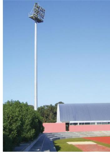
High Masts with lowering type lantern carriage & Rigid Platform are subject to inspection, testing & operation of winches in accordance with requirements of SHAWW (General Application) Regulations 2007, S.I. 299 of 2007.
