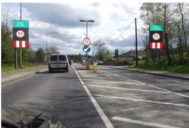
Gateway lighting using supplementary LED /150W Metal Halide lighting on double-headed column in central island. These should be hinged and socketed to allow the column to be lowered for Abnormal Loads
