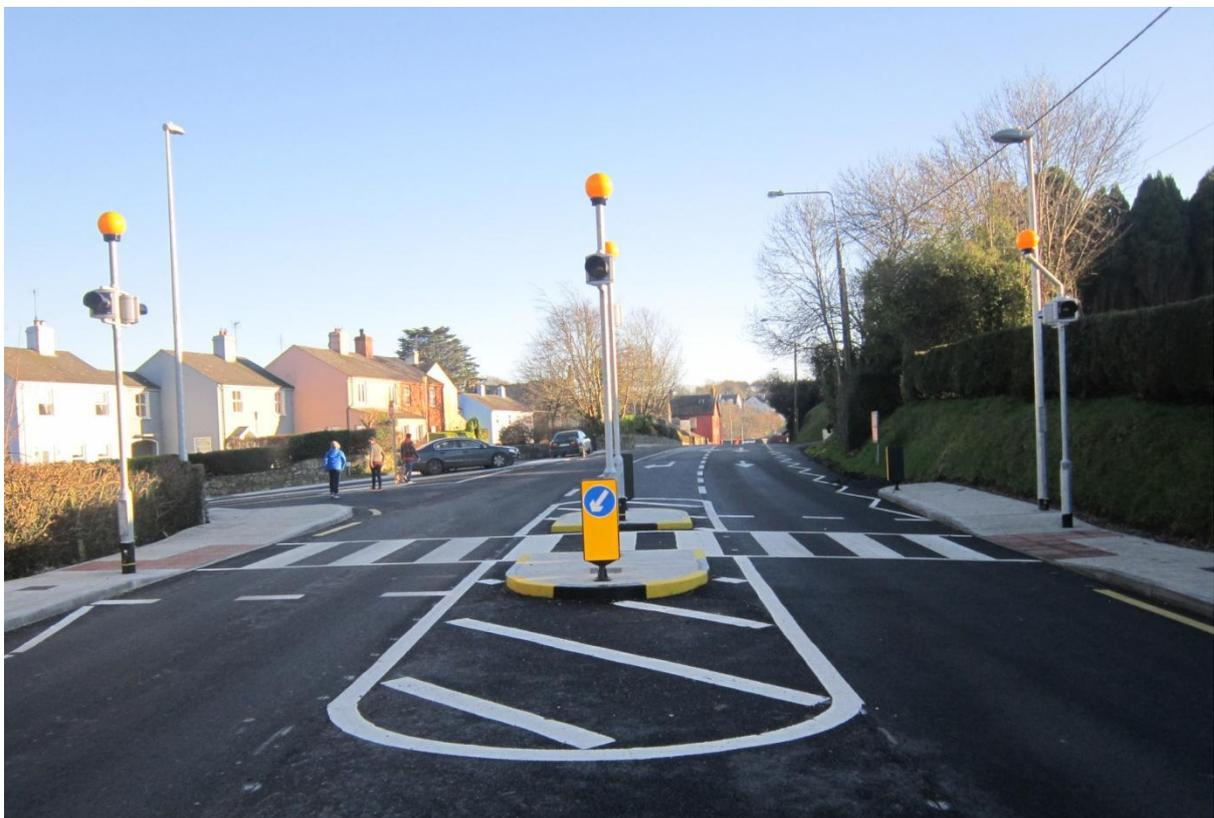
*Typical zebra crossing layout with special lights located on both diagonals.*
