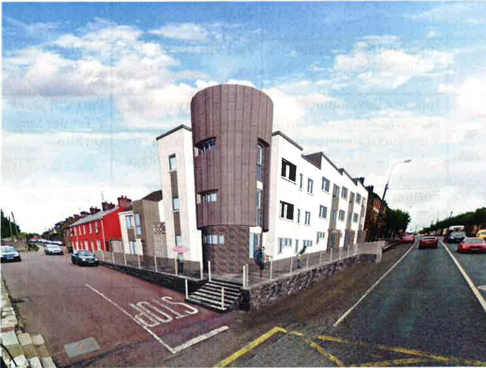
Housing at Oliver Plunkett Hill, Fermoy, County Cork
