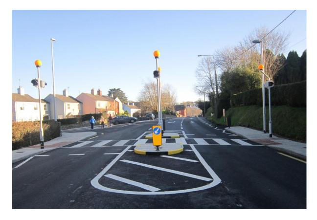
Typical zebra crossing layout with special lights located on both diagonals.
