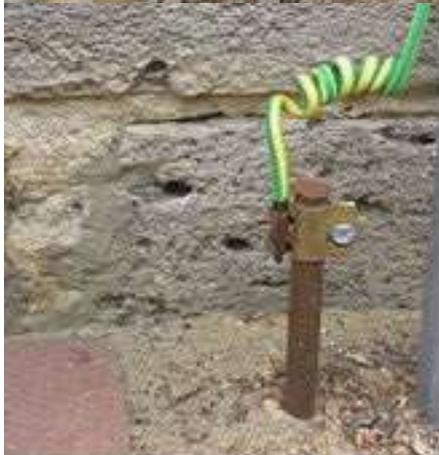
1.2m 16 sq mm galvanised steel earth rod and chamber for neutralising connection at minipillar
