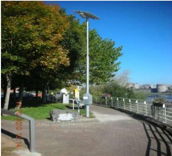
A further option combines solar power with wind power to typically output to a 35w LED Unit with integral Photocell & occupancy sensor , designed for instant start & delayed switch off after occupancy detection. In this option, the solar panel typically contributes 80w and the wind turbine 200w.
