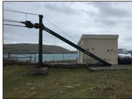
Plate 14.12: Island-side cableway machinery and line station
