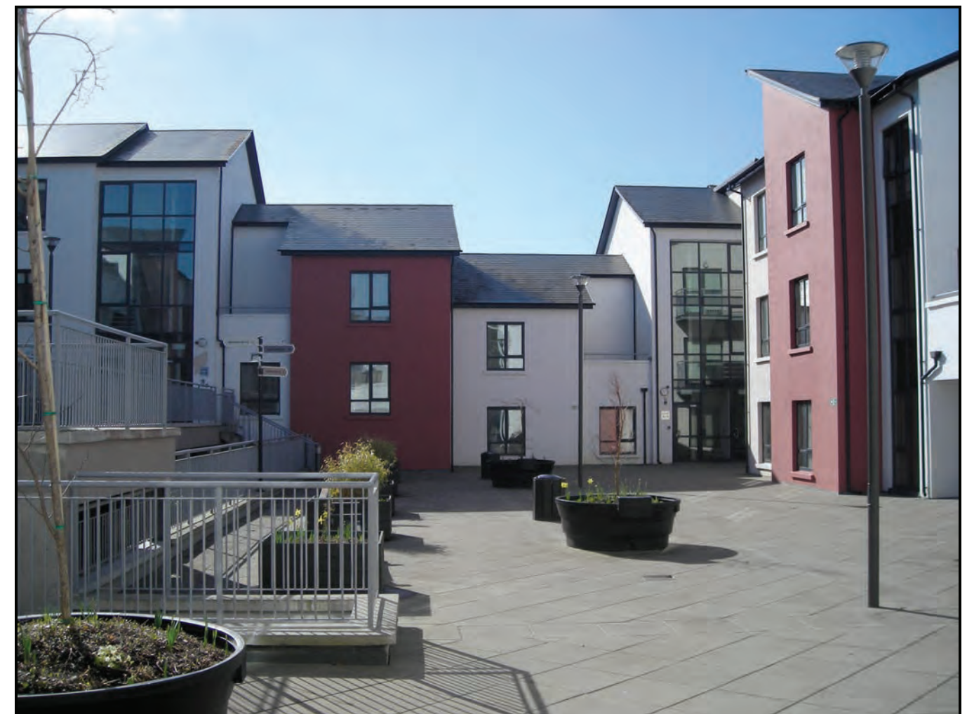
Courtyard Housing above parking level at Templegrove, Carr's Hill, Douglas
