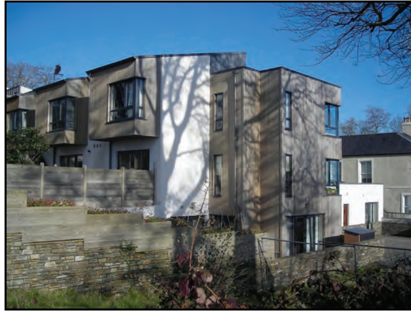
Housing with access from multiple levels on steep site at Woodville, Glanmire
