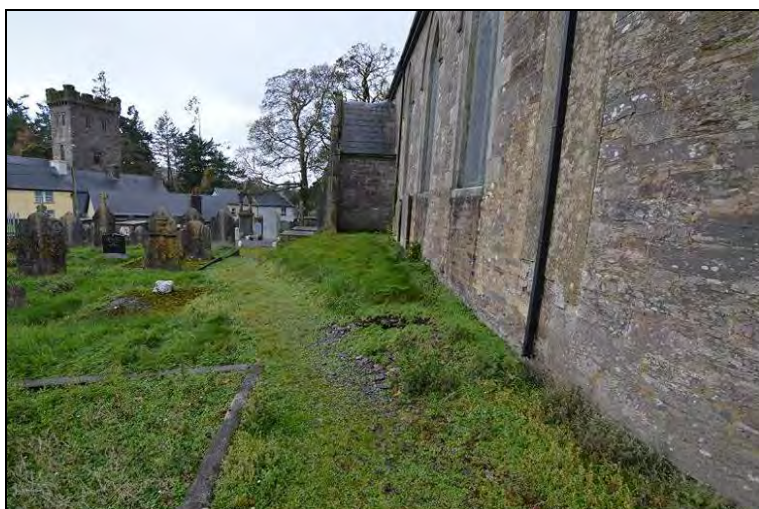
Photograph 9: View along the south elevation, showing the existing ground level against the church wall.
