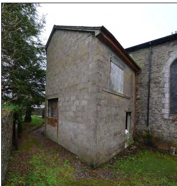
Photograph 13: The incomplete 1990s two storey concrete block replacement of the sacristy/robing room, viewed from the northwest.
