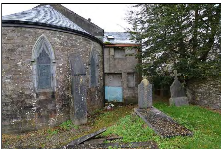
Photograph 11: The incomplete 1990s two storey concrete block replacement of the sacristy/robing room, viewed from the east.
