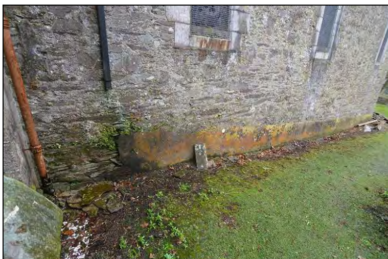
Photograph 15: Existing drain alongside the north wall, and cement render applied to the lower fabric.
