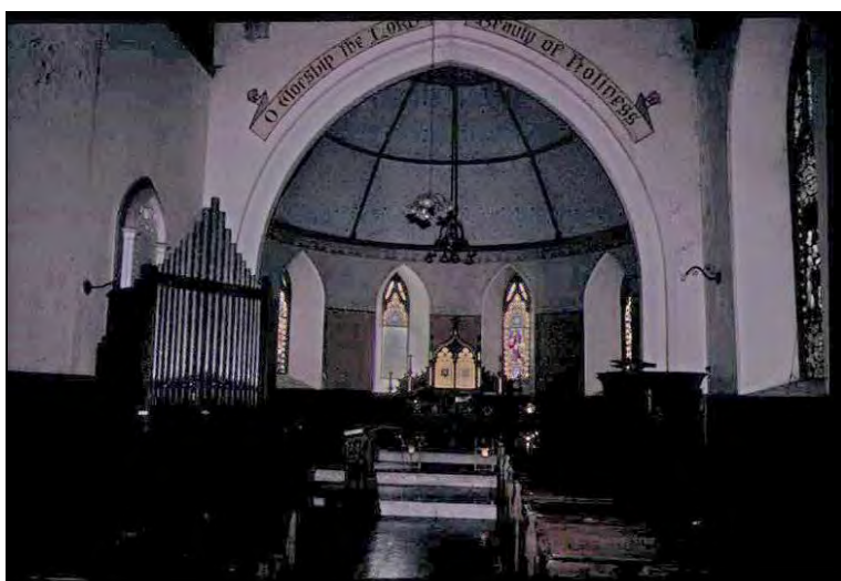
Photograph 16: View of the interior of the church body, looking southeast. Note the modern concrete floor, and the removed internal wall render – part of the significant 1990s works. The fabric, wall and floor surfaces of the Welland and Gillespie apse remains largely intact.
