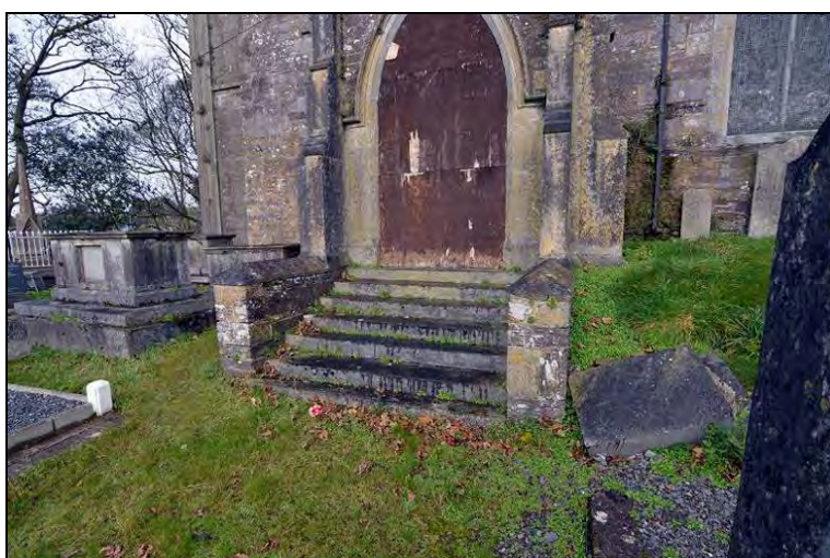
Photograph 8: View of the cut limestone steps to the porch. It is proposed to insert a wheelchair lift within the existing steps to give universal access to the porch and building.
