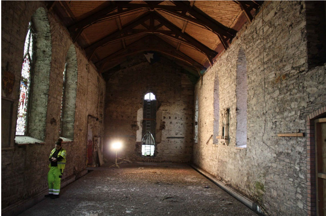
Main nave space looking west
