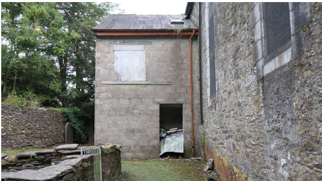
Existing extension – partially unfinished
