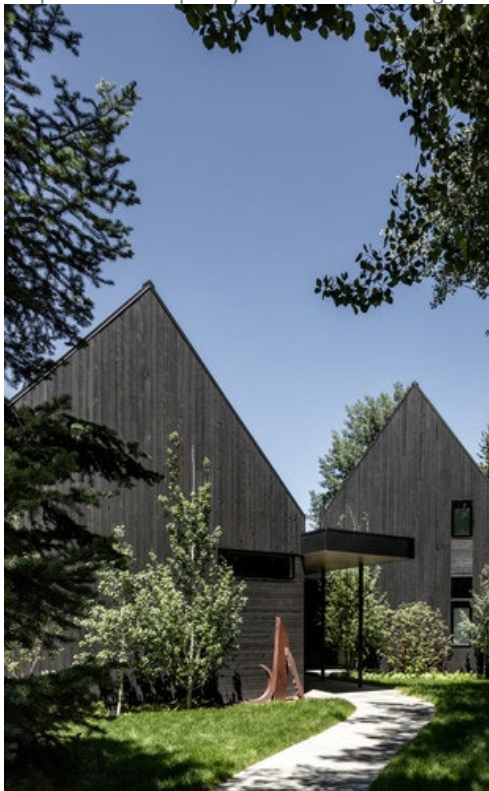
Example of timber larch cladding on walls and roof with concealed gutters and high-quality detailing
