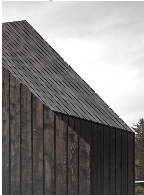
Example of timber larch cladding on walls and roof with concealed gutters and high-quality detailing
