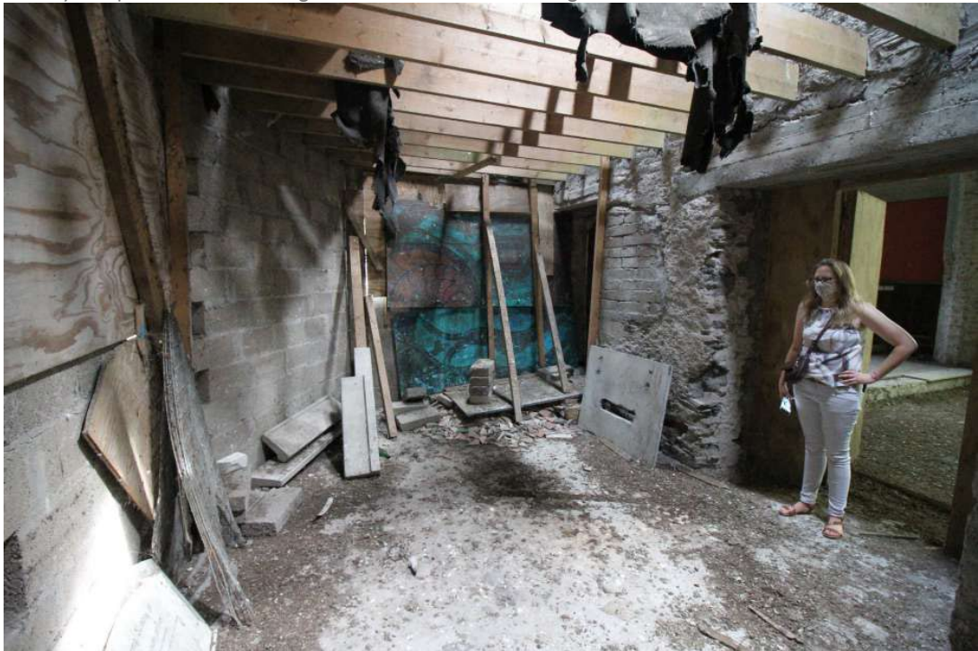
Partially completed Annex building looking East.
