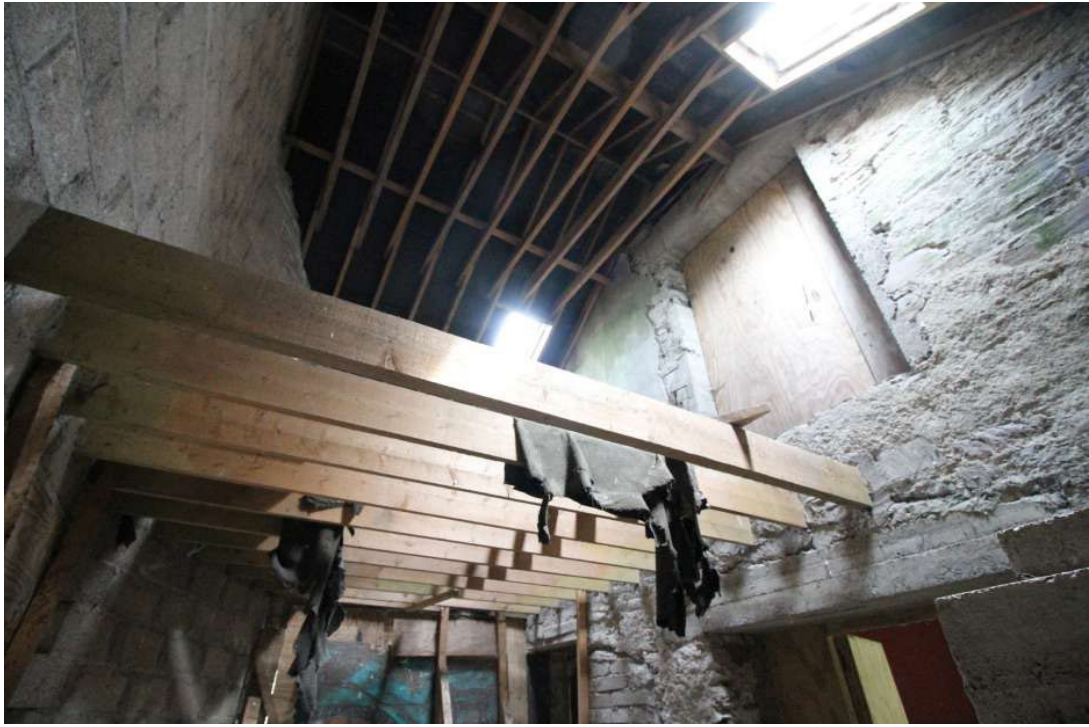
Partially completed Annex building with mezzanine access landing.
