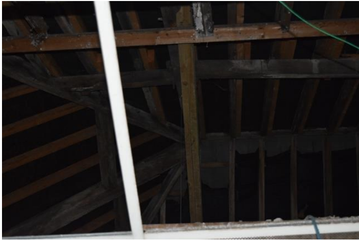
Image 22: Hipped roof timbers over Court Room.
