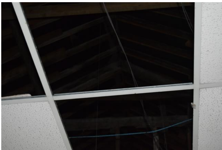
Image 23: Hipped roof timbers over Court Room.
