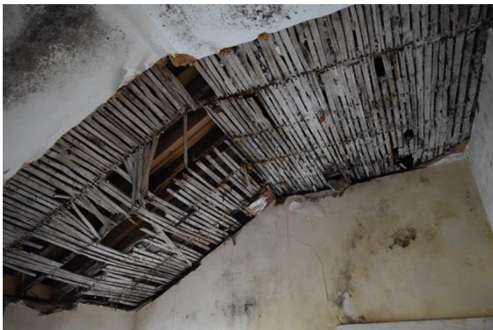
Image 27: Lath and plaster ceiling exposed in later extension. Poor condition.
