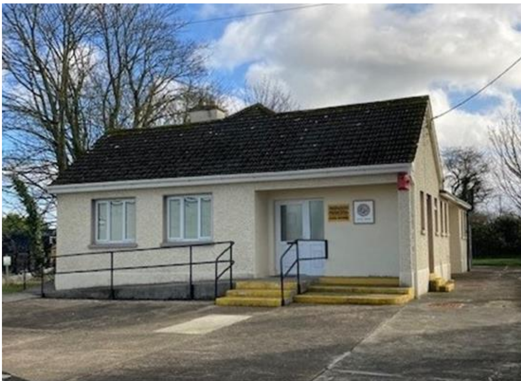
Figure 1. Photograph showing the HSE Building, Kilmallock Road, Charleville.
