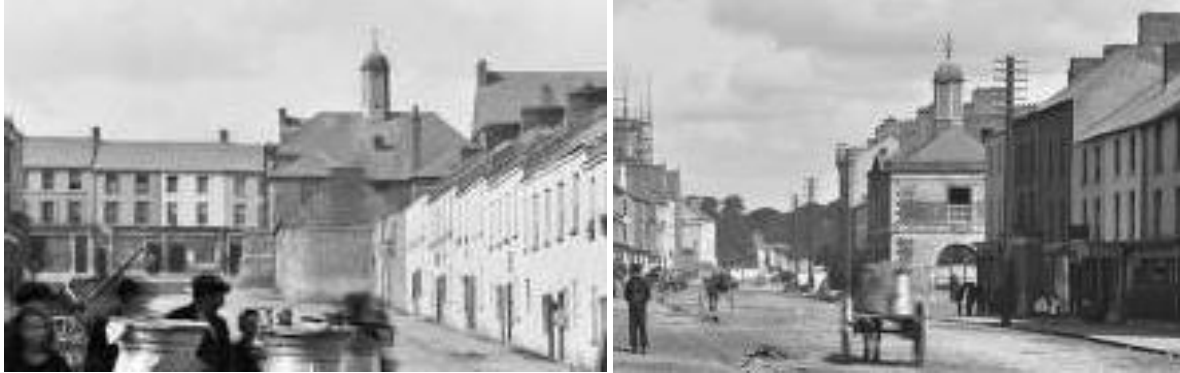
Figure 4: Photographs from the NLI's Lawrence Collection, dated c. 1880-1900, showing the cupola on the building in place
